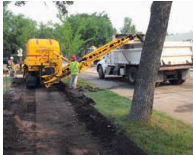
The GT-3400 trimmer's long discharge conveyor moves the trimmed material into haul units. It is trimming 1.9 meters (6.2 ft) wide on this project in Canada.
