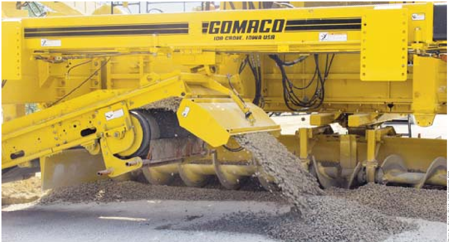
Ajax was placing stone over a geotextile fabric at a width of 32 feet (9.75 m) south of Grand Rapids, Michigan.
