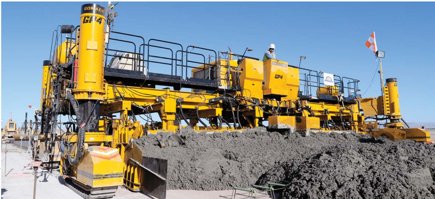
Paving the airport's new taxiway was completed in six days without any edge slump deficiencies and zero smoothness grinds. RGG United earned full payment for their paving on the project, as well as a six percent pavement bonus from the Federal Aviation Administration (FAA).
