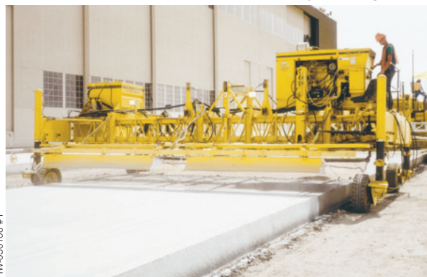
A T/C-400B applies the cure to the slab.
