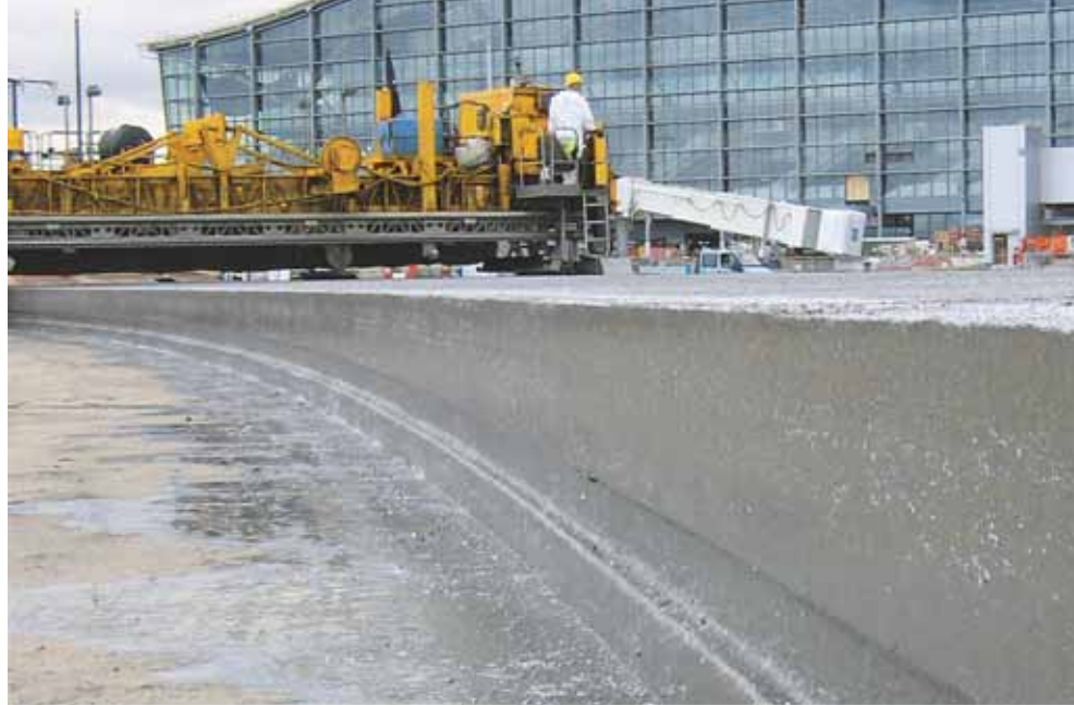
The new pavement was designed with a structural strength high enough to accommodate the largest aircraft, including the Airbus A380.
