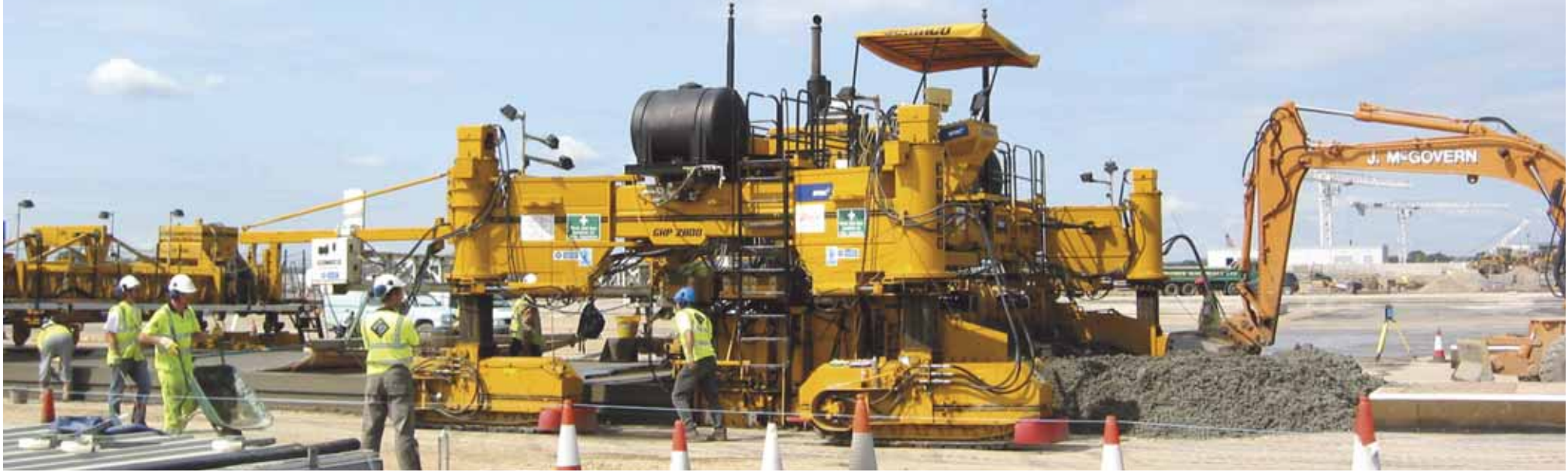
A GOMACO four-track GHP-2800 slipforms concrete on the new Terminal 5 (T5) at London Heathrow Airport.
