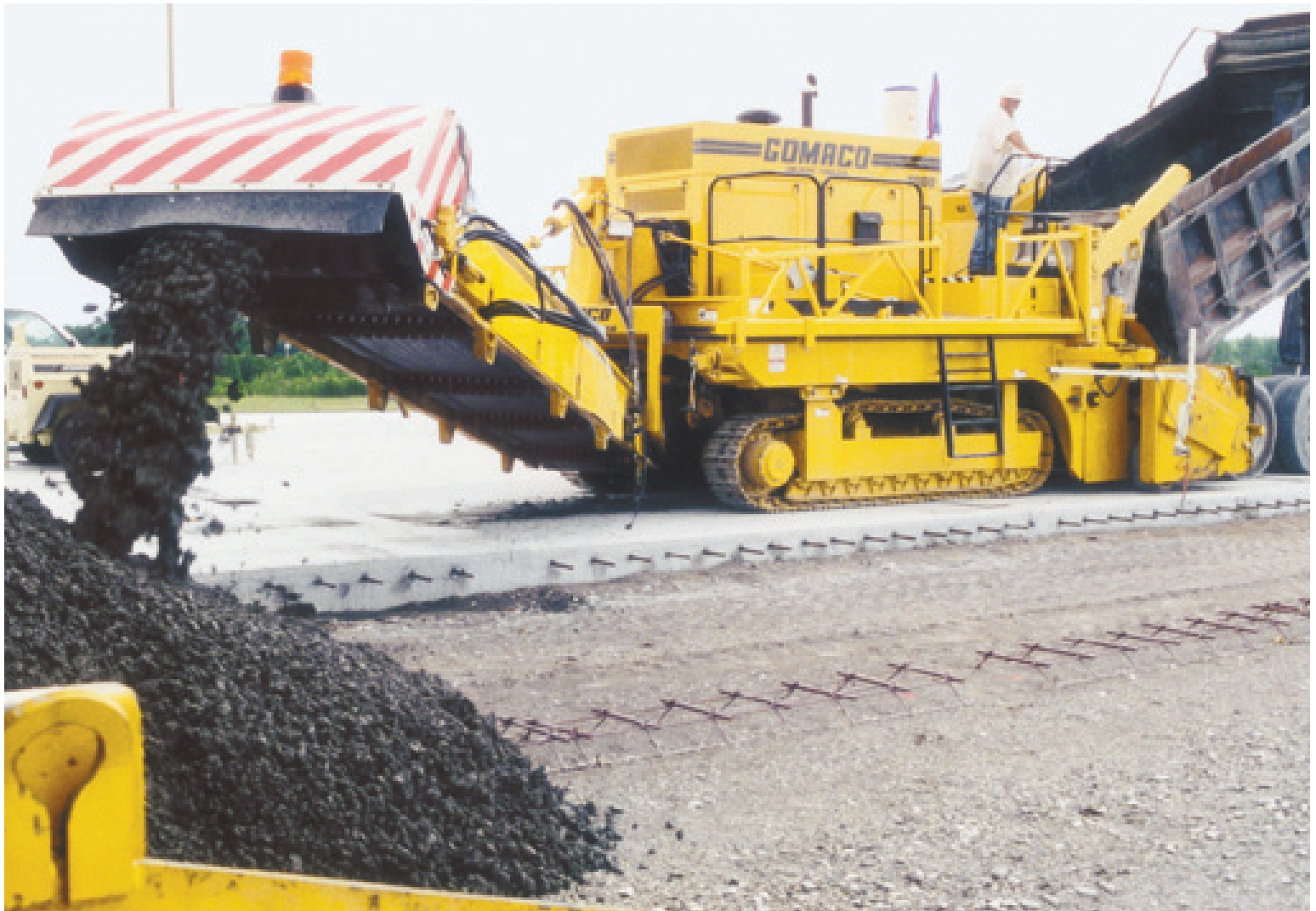
A GOMACO 9000 placer was used to place concrete in front of the paver on a majority of the project.
