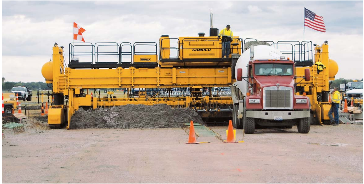
Paving production with the GOMACO GP-4000 averaged 400 cubic yards (305.8 m 3 ) per hour. A second batch plant had to be utilized to keep up with the paver's production while slipforming 37.5 feet (11.4 m) wide.
