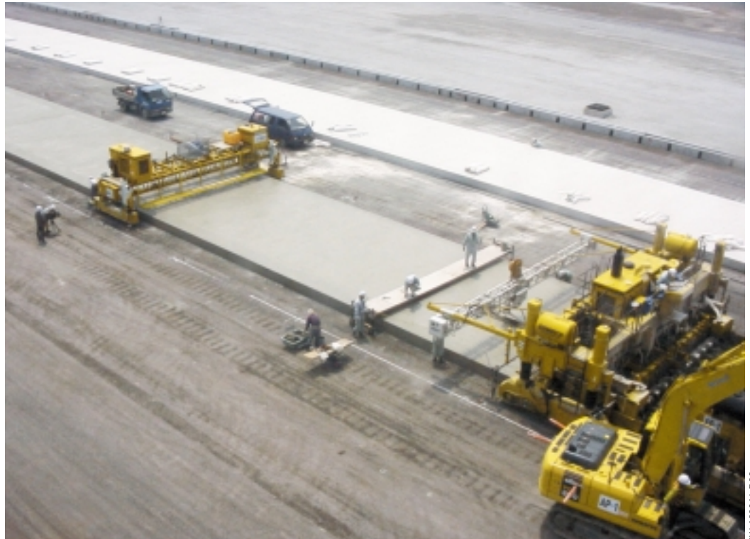
A T/C-400 follows behind the paver applying a transverse tine to the new runway.
