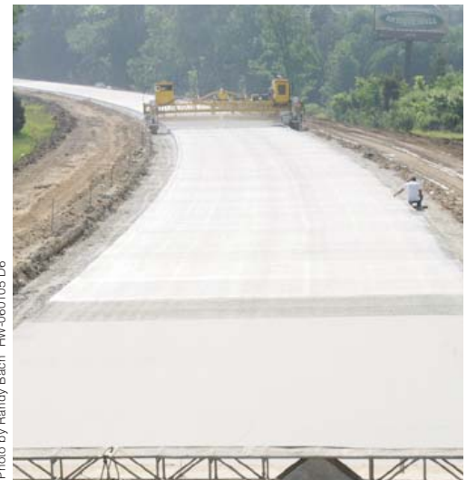
The GHP-2800 with IDBI (left) slipforms underneath a bridge overpass.
