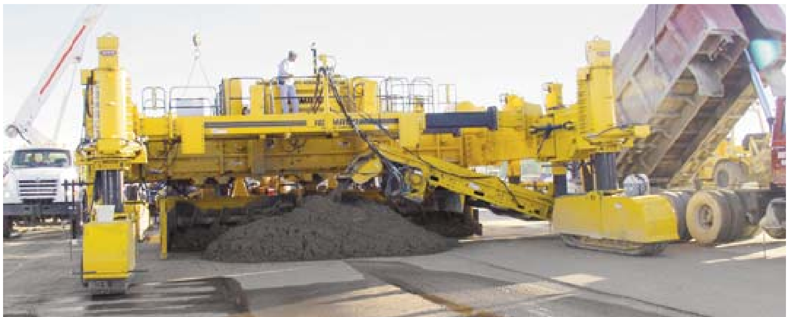
The PS-4000 easily handled the one inch (25 mm) slump concrete and helped Ajax achieve record-setting production.
