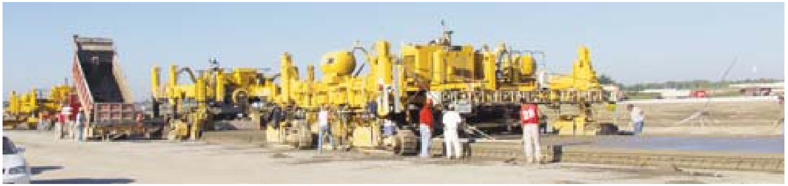
The GP-3000 paver follows the PS-4000 and PS-60 placer/spreaders on the Detroit Metro Airport.
