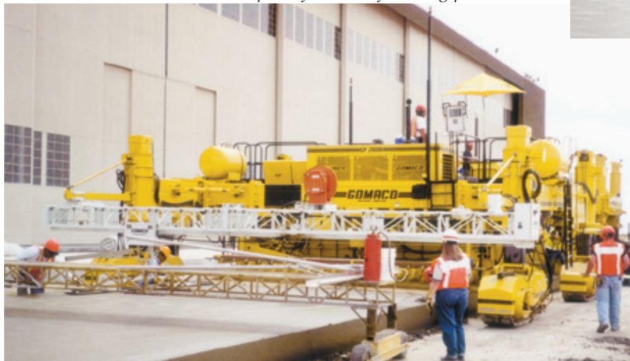
An advantage of a stringless job site is how much it opens up the site.
