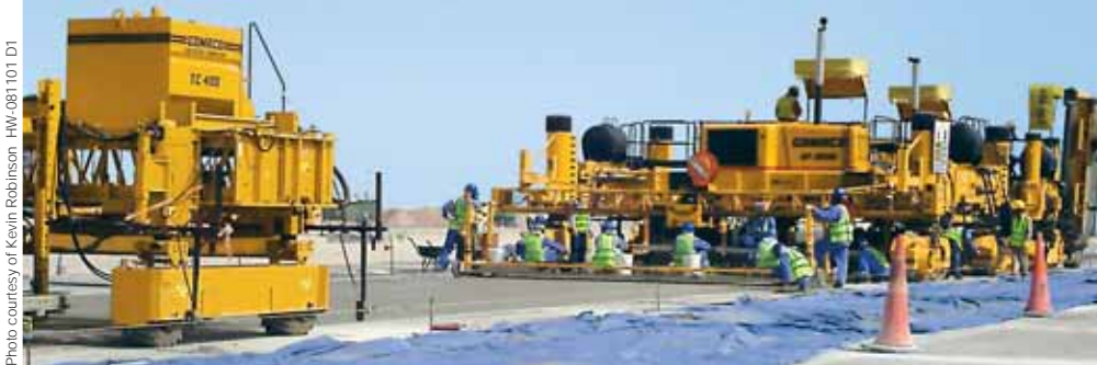
A GOMACO PS-2600 placer/spreader, four-track GP-2600 paver and T/C-400 texture/cure machine at work on the New Doha International Airport in Qatar.
