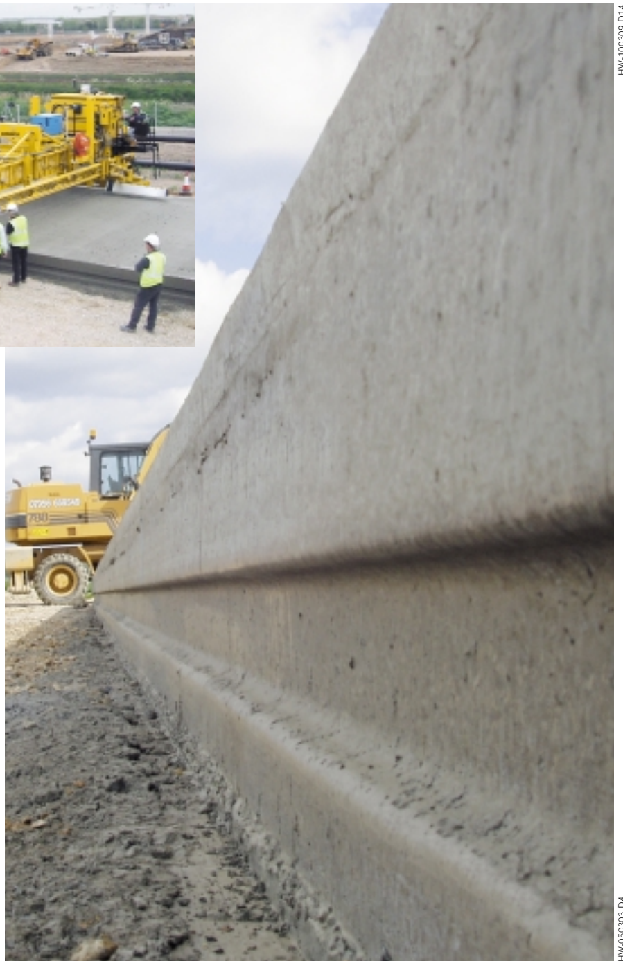
Work is currently underway on the T5 project at London Heathrow Airport. A GHP-2800 is slipforming slabs 21.7 inches (550 mm) thick. Two Compactor-brand batch plants are providing concrete for the project.
