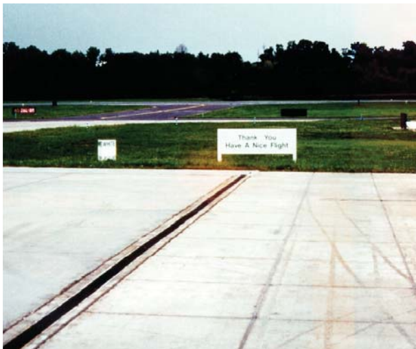
Figure 3. Photo of the completed concrete overlay at Spirit of St. Louis Airport in 1994.
