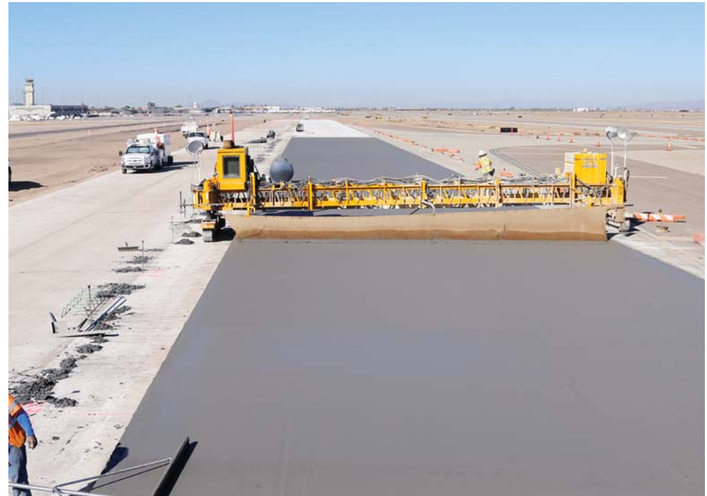
Wider-width airport paving is just one of the applications the GP4 was designed to pave. At the Phoenix-Mesa Gateway Airport, the GP4 was slipforming 37.5 feet (11.4 m) wide and 16.5 inches (419 mm) thick.
