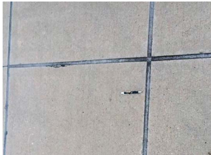
Figure 4. Current pavement condition (June 2015).
