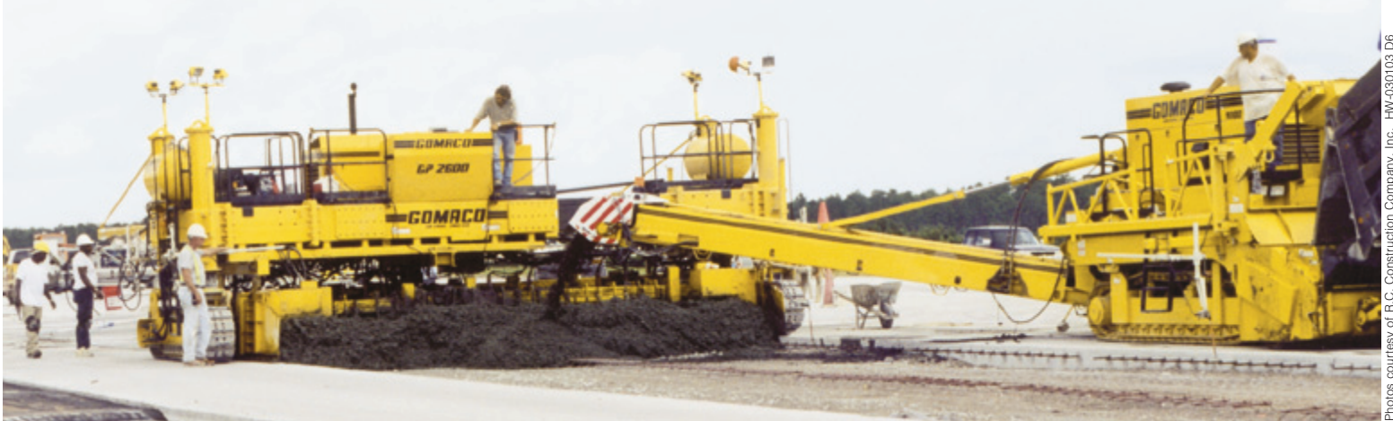
Photos courtesy of R.C. Construction Company, Inc. HW-030103 D6
