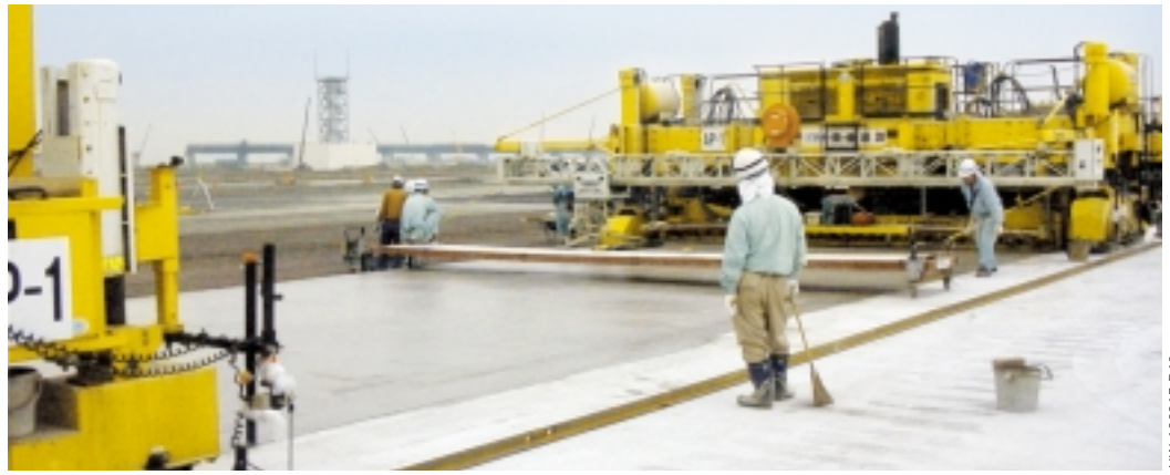
Toa's GHP-2800 slipforms on the new runway. They're paving 24.6 feet (7.5 m) wide and thickness varied between 16.5 to 18.1 inches (420 to 460 mm).
