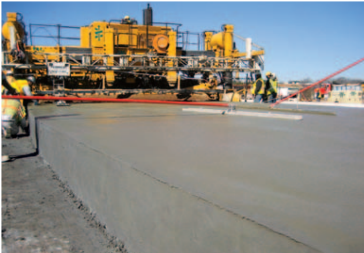
The new Taxiway V is 130 feet (39.6 m) wide, 4200 feet (1280 m) long and 20 inches (508 mm) thick.
