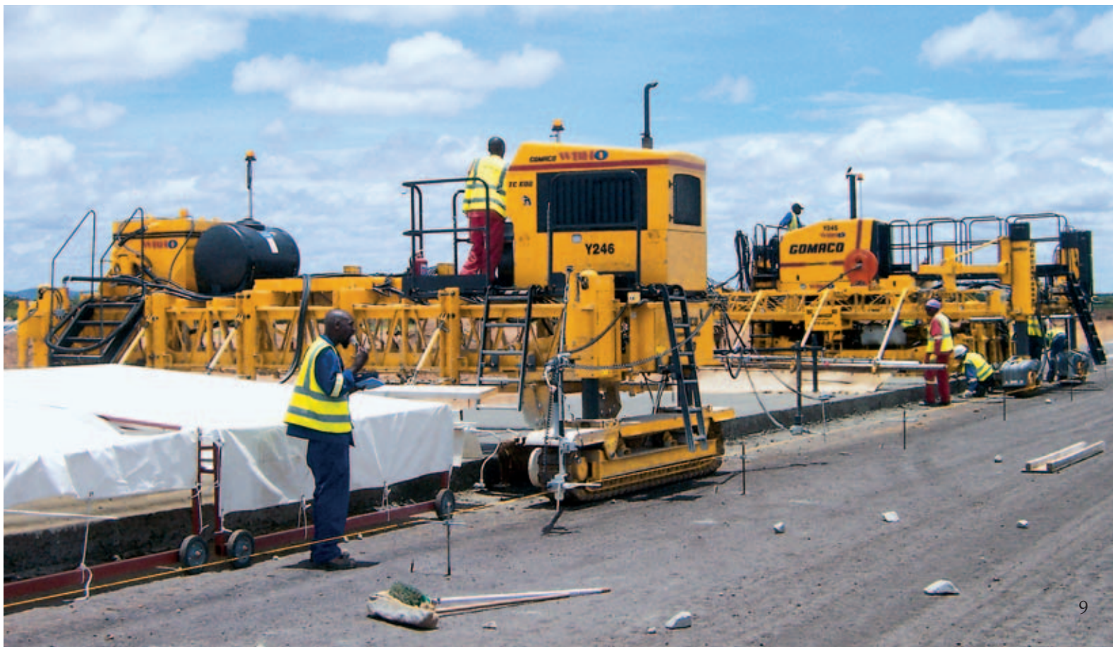
The new runway had to be protected from Botswana's extreme heat. A GOMACO T/C-600 applied a white spray cure directly behind the paver and tenting structures were used to shade the concrete to keep it from curing too fast.
