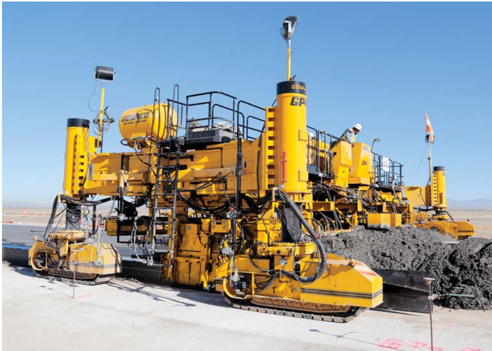
RGG United was able to utilize their existing attachments and sensors from their GOMACO GP-4000 paver on their new GP4 with G+ control system.
