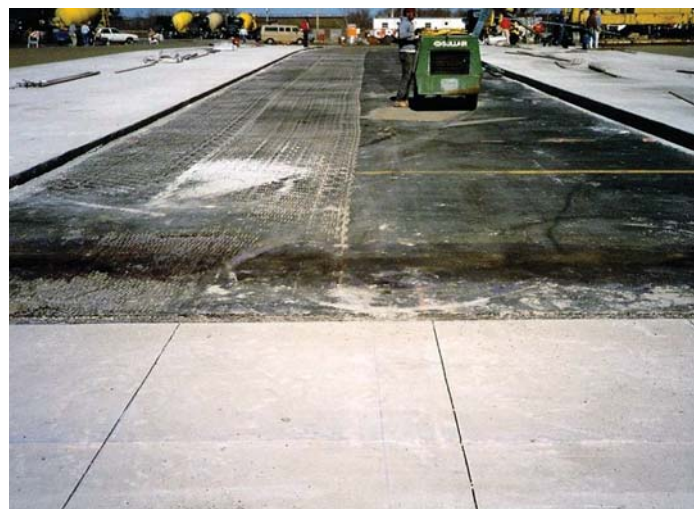
Figure 2. Photo from original construction of the concrete overlay at Spirit of St. Louis Airport in 1994.
