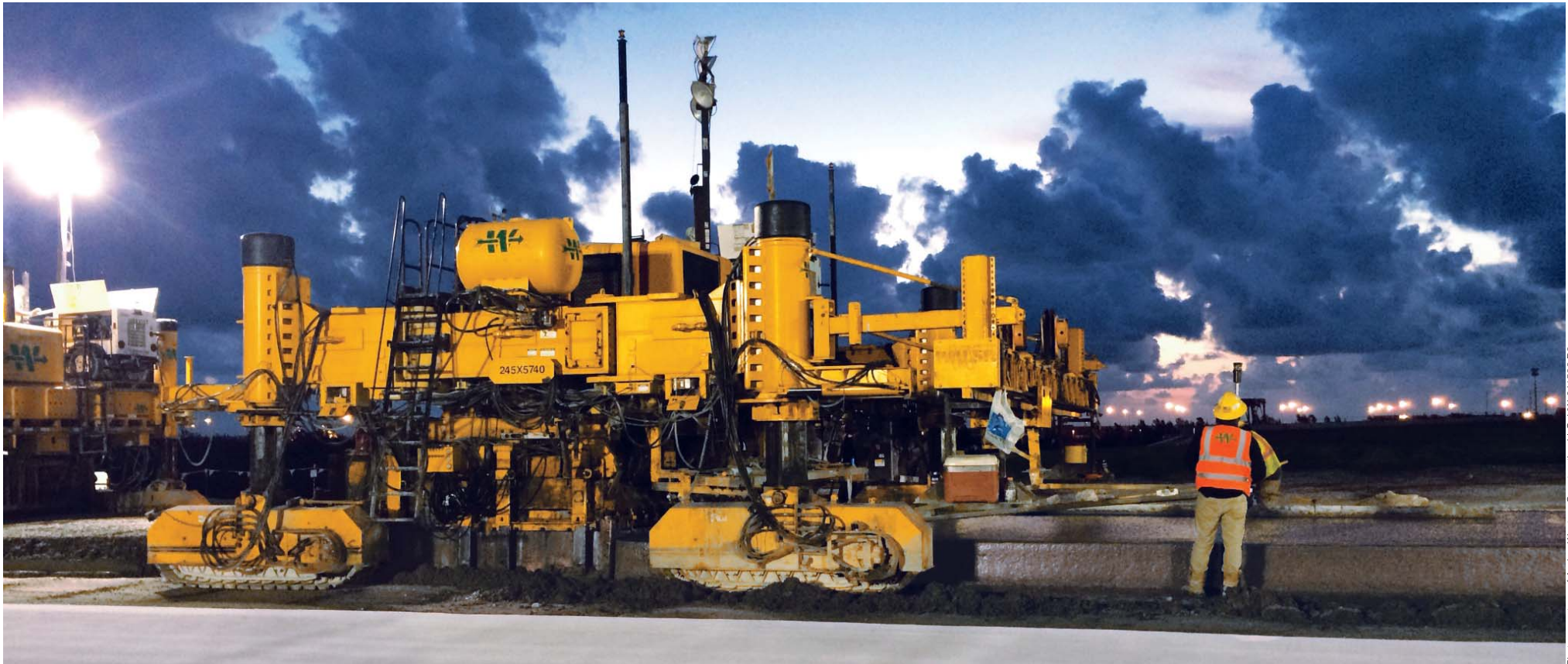
Photos courtesy of Archer Western Construction LLC HW-041522 D2
