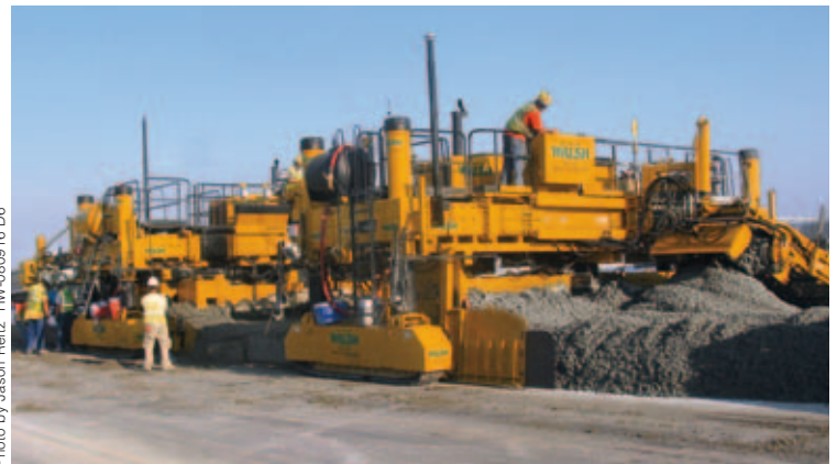
Photo by Jason Reitz HW-080916 D6 A GOMACO PS-2600 placed and spread the concrete in front of the two-track GHP-2800 slipform paver.
