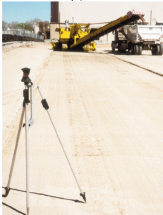
A prism set on the trimmed grade is used to measure the accuracy of the 9500's cut.
