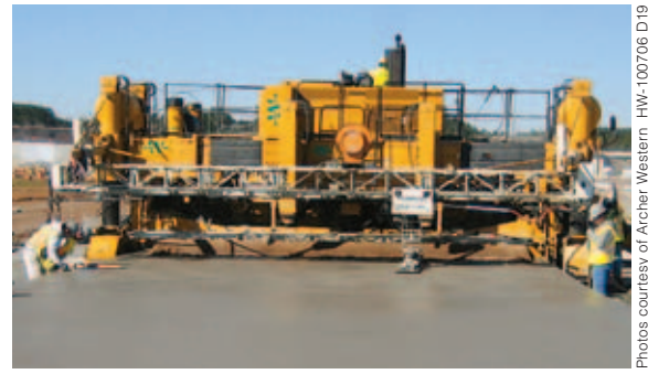
Photos courtesy of Archer Western HW-100706 D19
