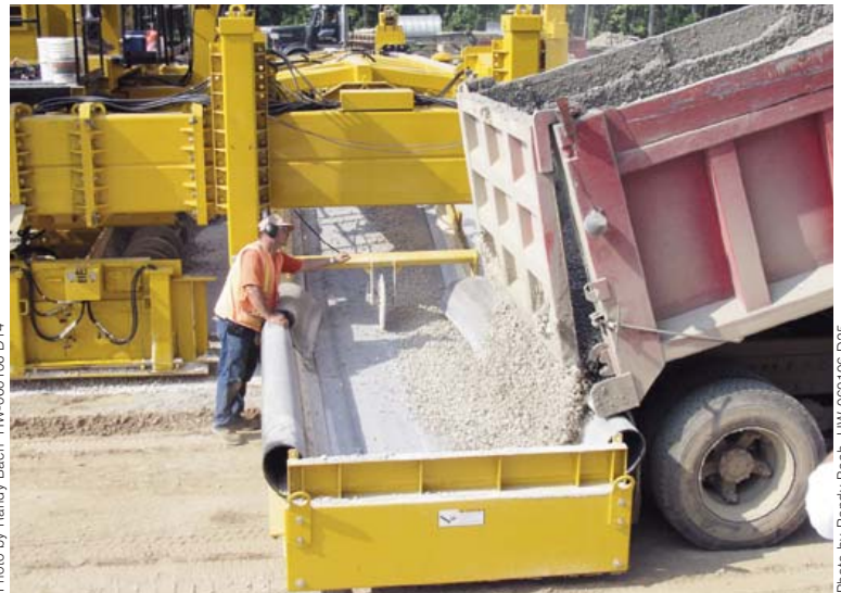
Gravel trucks dump their load of stone directly onto the conveyor of Ajax's PS-4000.
