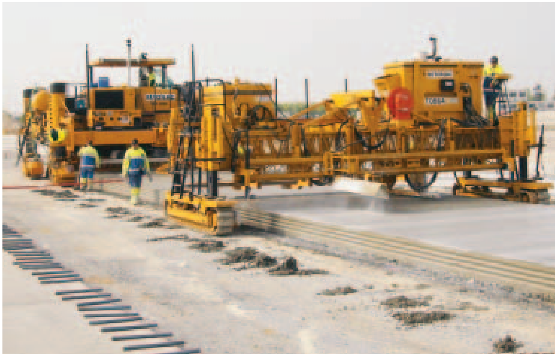
Betonac’s GOMACO paving train completed 34 paving passes on the airport project. Each pass was 300 meters (984 ft) long, five meters (16.4 ft) wide and 400 mm (15.7 in) thick.
