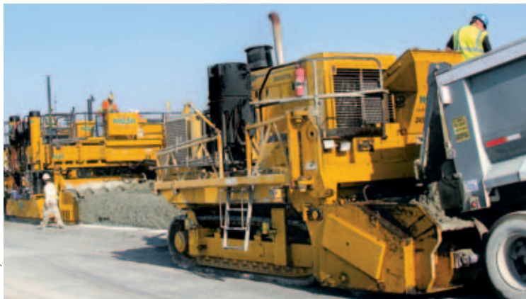
Photo by Jason Reitz HW-080917 D1 Thirty-nine end-dump trucks were needed to keep the average paving production at 618 cubic yards (472 m 3 ) per hour.
