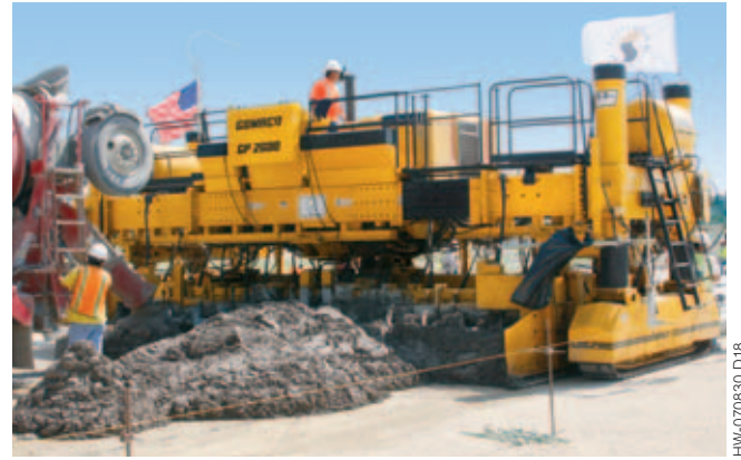
The 650 flex concrete mix was dumped directly on the grade in front of the new GP-2600 two-track paver.
