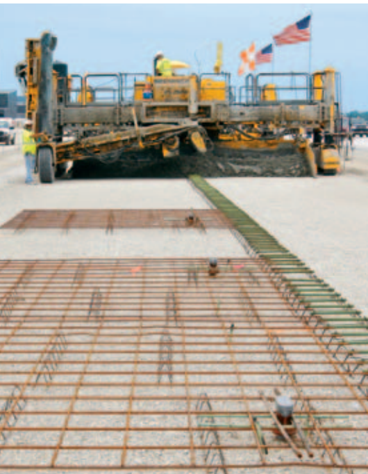
A 9500 prepares grade ahead of the GOMACO paving train.
