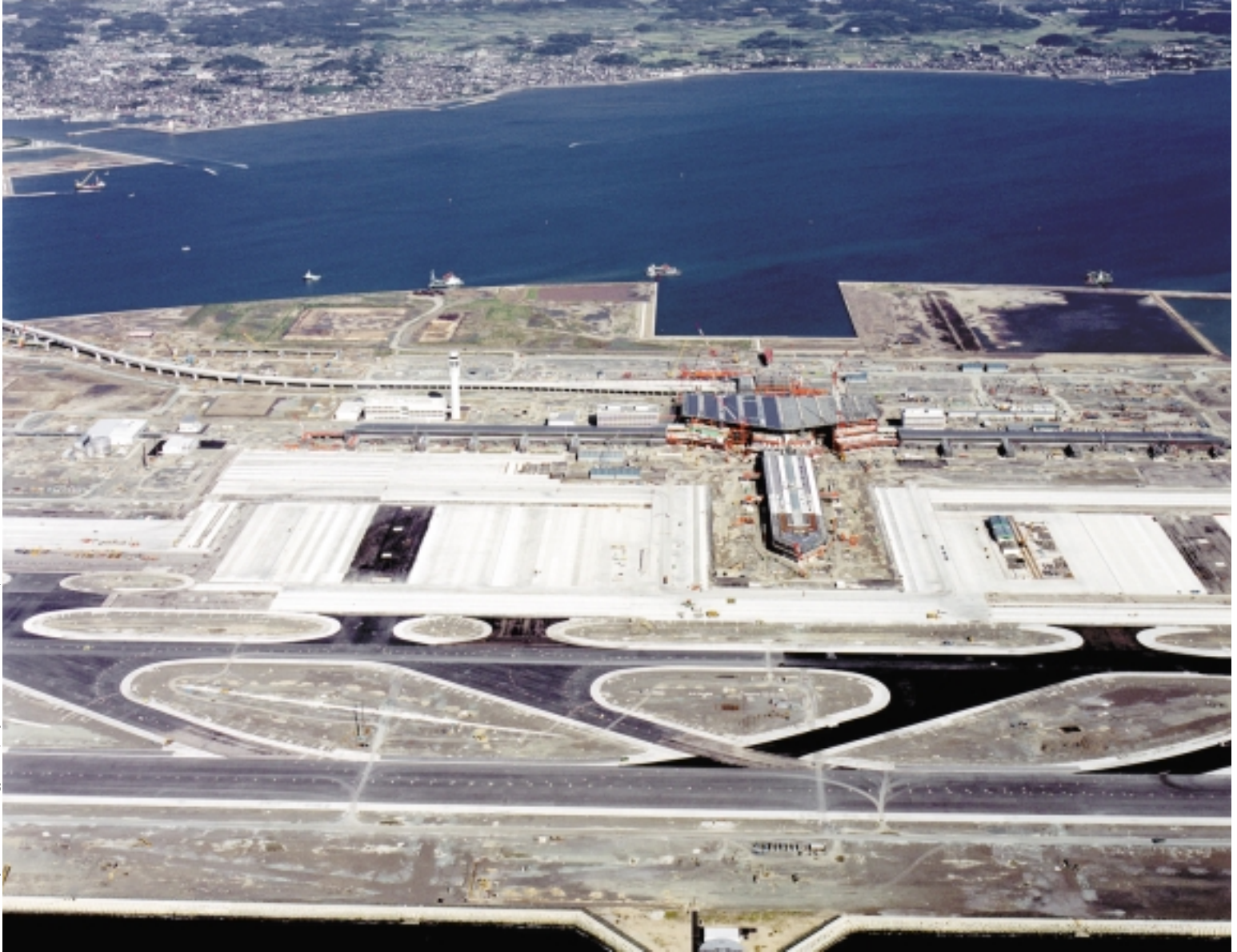
Photos courtesy of Toa Doro Kogyo Company, Ltd., and Taisei Rotec Corporation. HW-120302 D17
