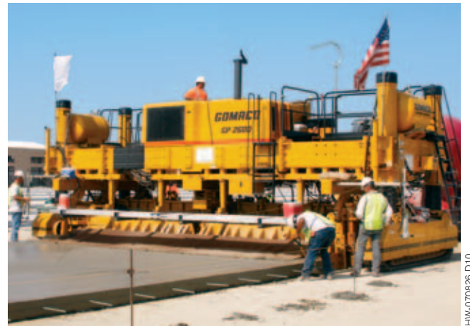
Straight edge requirements allowed only a 0.25 inch (6 mm) deviation in 16 feet (4.9 m).
