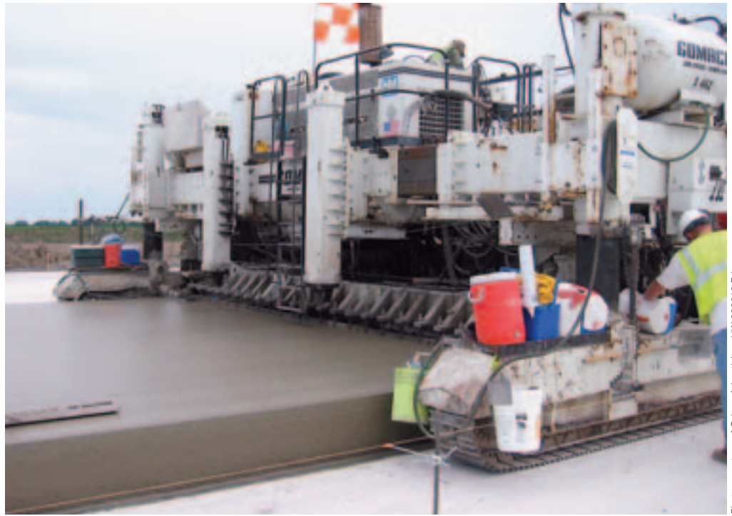
The mix was so consistent that no edge slump boards were required and bull-floating behind the paver was minimal.
