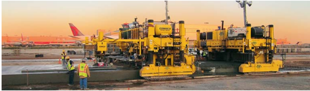
The sun goes down at Hartsfield-Jackson Atlanta International Airport as Archer Western slipforms another 25 foot (7.6 m) wide paving pass for the airport's new apron.
