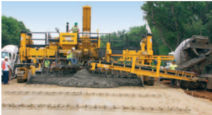
The GP-2600 has a front-mounted conveyor system to help with the project’s tight conditions.
