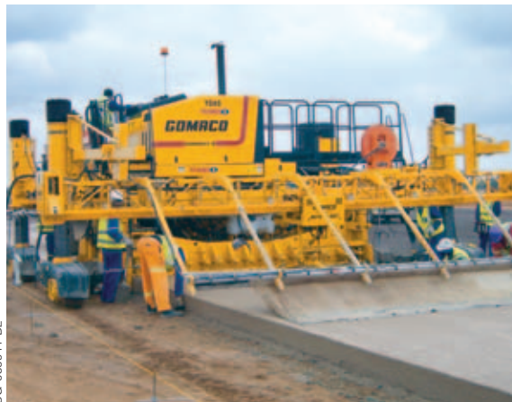
Paving passes were 4.5 meters (14.8 ft) wide and 320 millimeters (12.6 in) thick.
