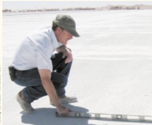
Ken Tippie checks for edge slump.
