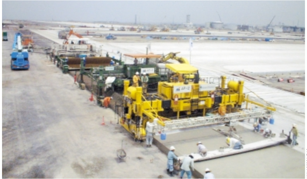
Taisei purchased the GHP-2800 paver specifically for this project. They wanted a paver that could meet the strict specifications on this first commercial airport slipforming project.
