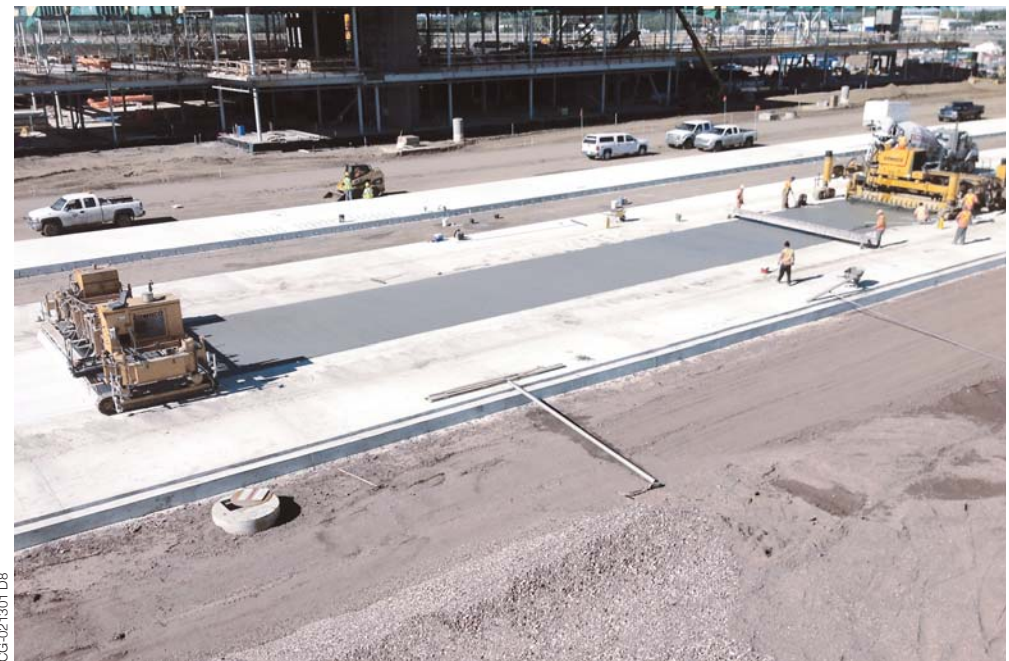
CG-021301 D8 The Commander III slipformed the new apron in six paving passes. Each pass was 6.1 meters (20 ft) wide and 380 millimeters (15 in) thick.
