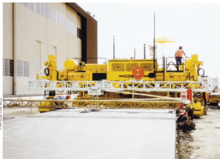
This Corps of Engineers’ project has strict guidelines on concrete thickness, smoothness and finishing.
