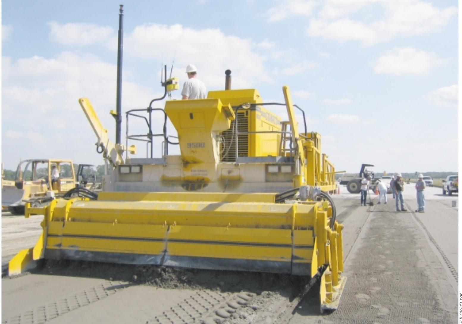
The 9500, equipped with the stringless technology, trims the cement-treated base (CTB) down to the six inch (152 mm) specification.
