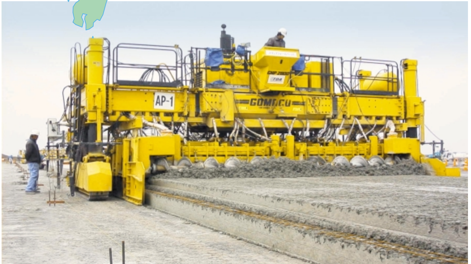
Concrete is spread to a thickness of 11.6 inches (295 mm), mesh is laid on top and a second placer/spreader adds another 4.9 inch (125 mm) thick layer.
