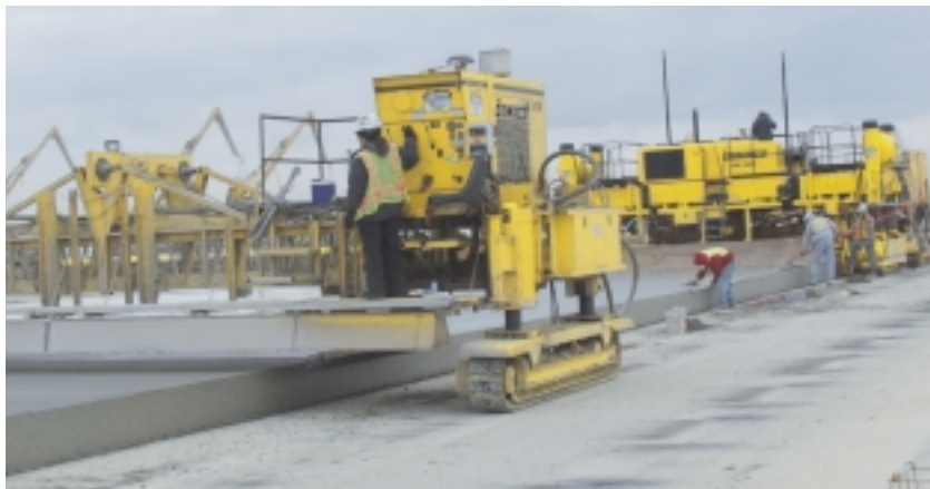
A T/C-600 texture/cure machine follows behind the paver.
