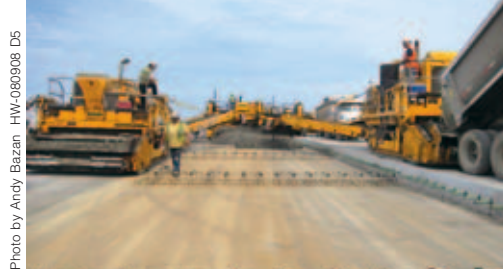
Photo by Andy Bazan HW-080908 D5 Two GOMACO 9500s placed concrete on grade in front of the PS-2600 which was placing and spreading the concrete in front of the GHP-2800 paver.
