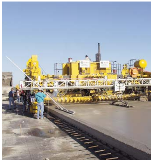
The GHP-2800 paver slipforms a pass on the Detroit airport.
