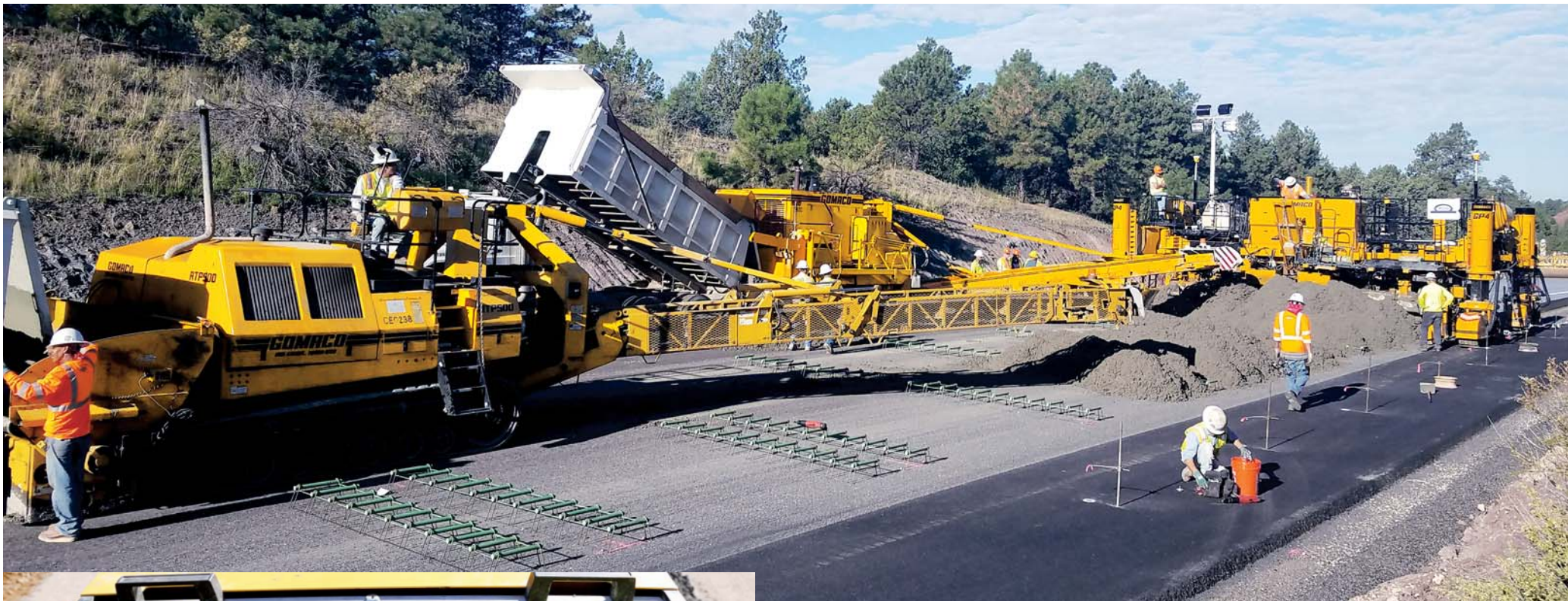
A GOMACO RTP-500 and 9500 concrete placer work in front of the GP4 paving 22 feet (6.7 m) wide on the I-40 Devil Dog project replacing five miles (8 km) of the interstate's eastbound lanes.
