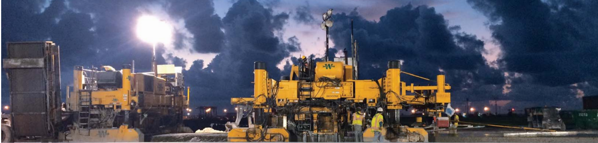
Archer Western Construction LLC slipformed the new 8000 foot (2438 m) southern runway with their GOMACO PS-2600 placer/spreader, GHP-2800 paver, and T/C-600 texture/cure machine.
