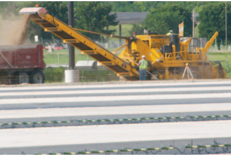
A 9500 prepares grade ahead of the GOMACO paving train.
