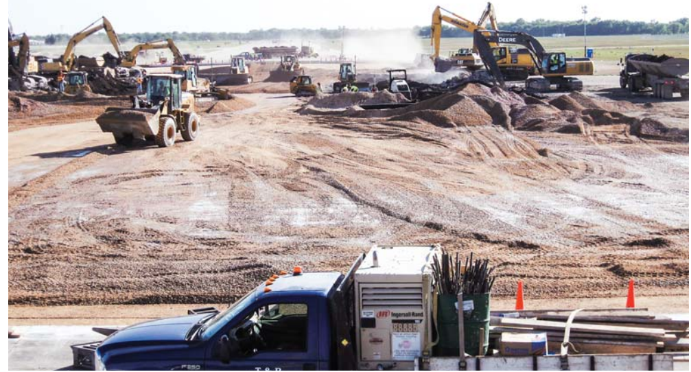
Thirty pieces of equipment and over 80 trucks were utilized to demolish and remove the existing runway and subbase which was approximately 42 inches (1067 mm) in depth.
