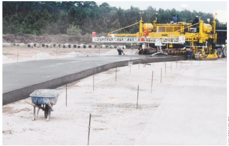
A GP-2600 and GP-2000 were used to slipform the 8000 feet (2438 m) long and 150 feet (46 m) wide runway.
