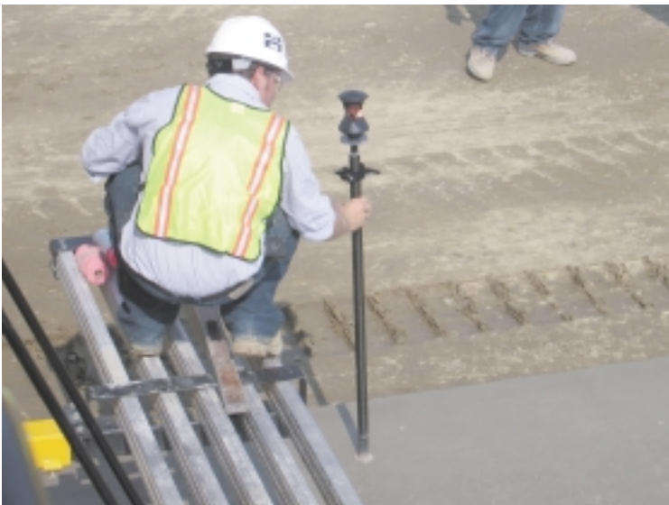
A worker uses a prism to conduct an as-built check behind the paver and ensures correct concrete placement on the project.
