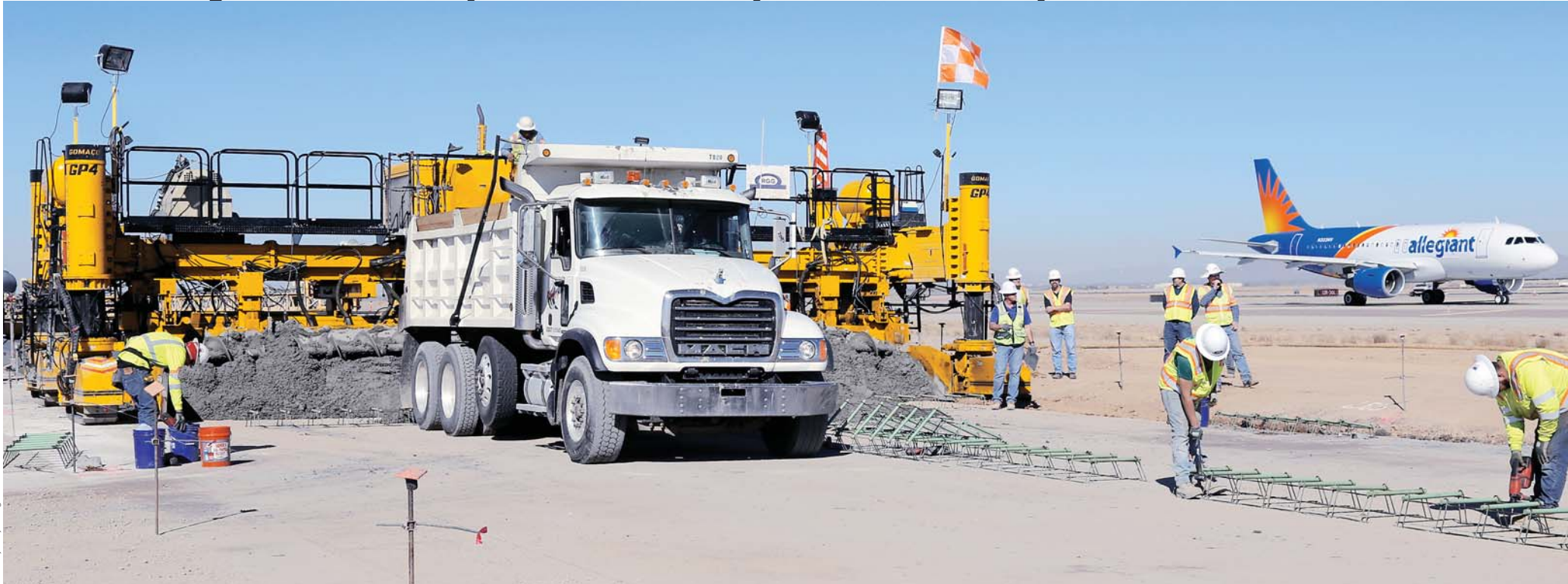
The new GP4 is capable of paving widths up to 40 feet (12.2 m) wide and is the ideal paver for airport work when exacting smoothness and edge slump requirements must be met using difficult concrete mix designs.
