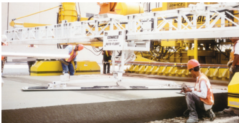
A GOMACO Auto-Float® was part of the slab finishing process.
