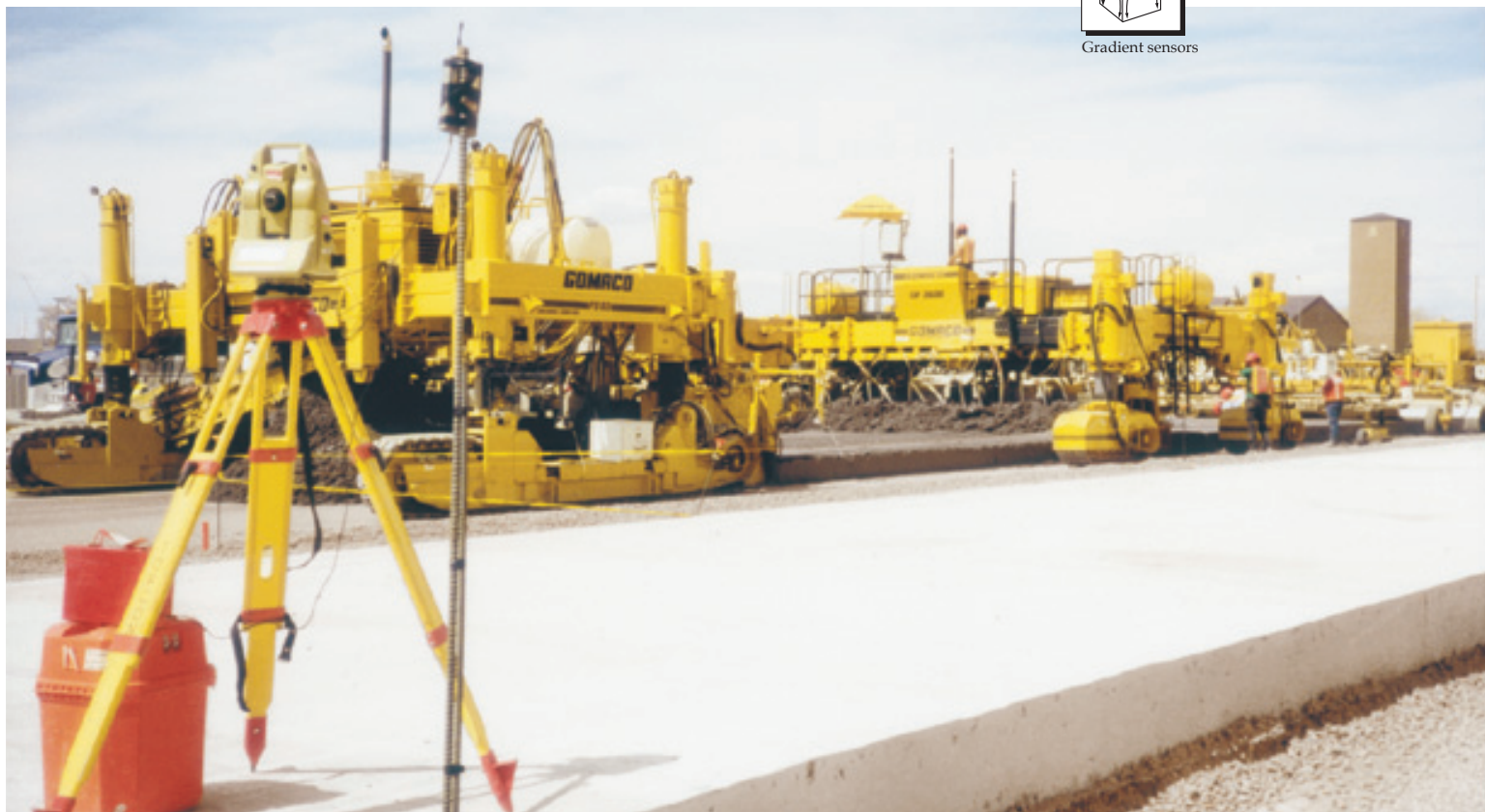
Tracking information from the total stations is relayed back and forth by radio signals to the Command Center.
