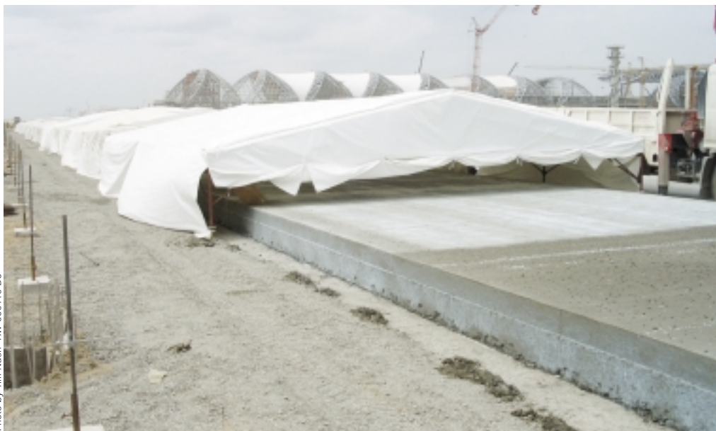
The width of the new slabs varies between 16.4, 18 and 19.7 feet (5, 5.5 and 6 m) wide. All of the slabs are 17.7 inches (450 mm) thick.
