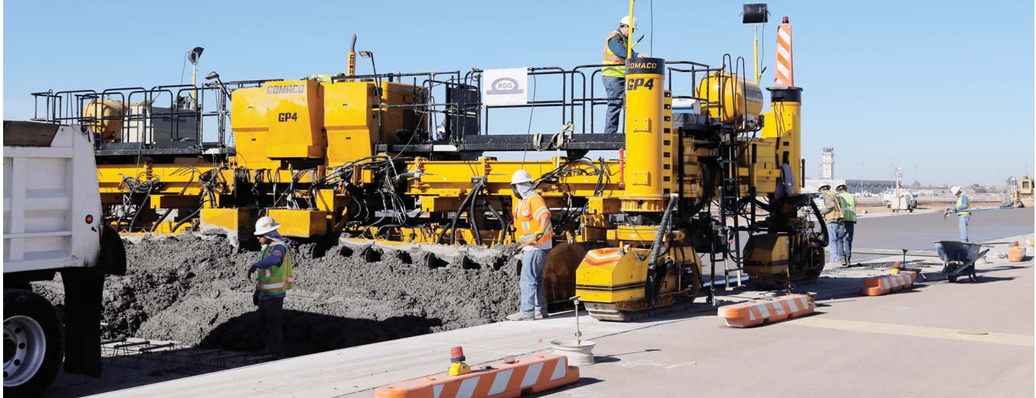
The control tower for the Phoenix-Mesa Gateway Airport can be seen behind the GP4 paver as it slipforms the new 3500 foot (1067 m) long, 75 feet (22.9 m) wide curbside-rated aircraft taxiway.
