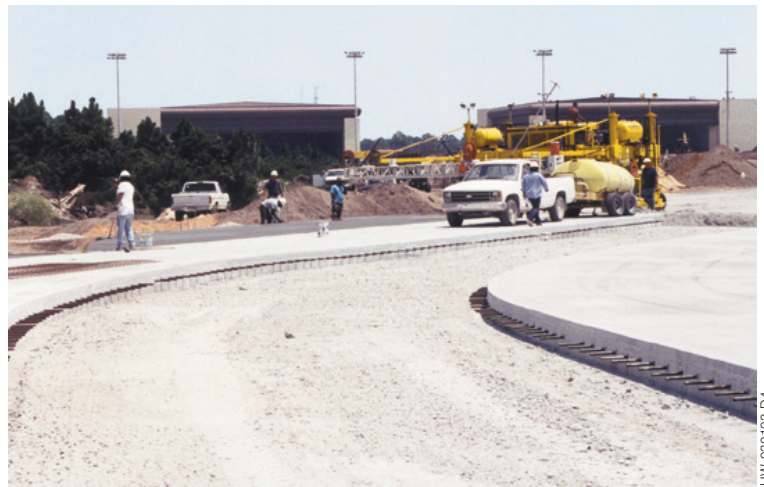
Holes were drilled into the edge of the slab and dowels were manually inserted and epoxied.
