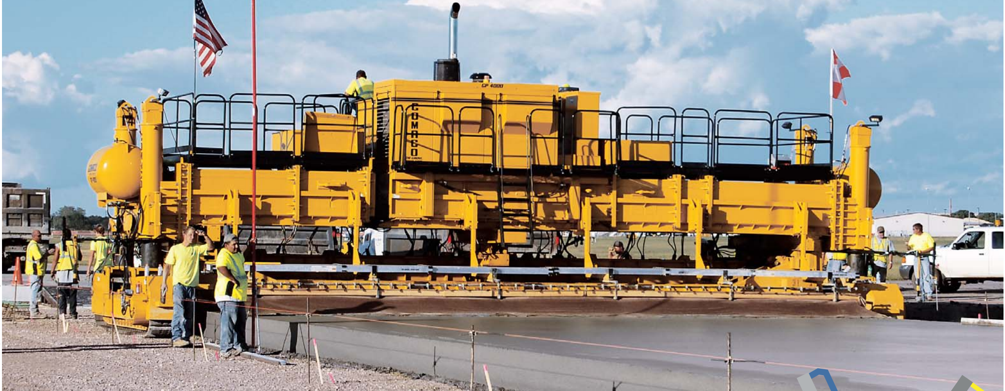
The intersection between the two major runways at the Sioux Falls Airport was removed and replaced in just two weekends by T&R Contracting Inc.
