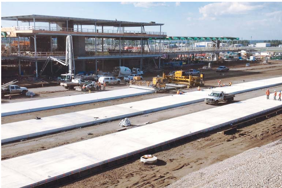
CG-021301 D6 Proform Concrete Services Inc., used their GOMACO four-track Commander III to slipform an apron next to the new terminal building at the airport.
