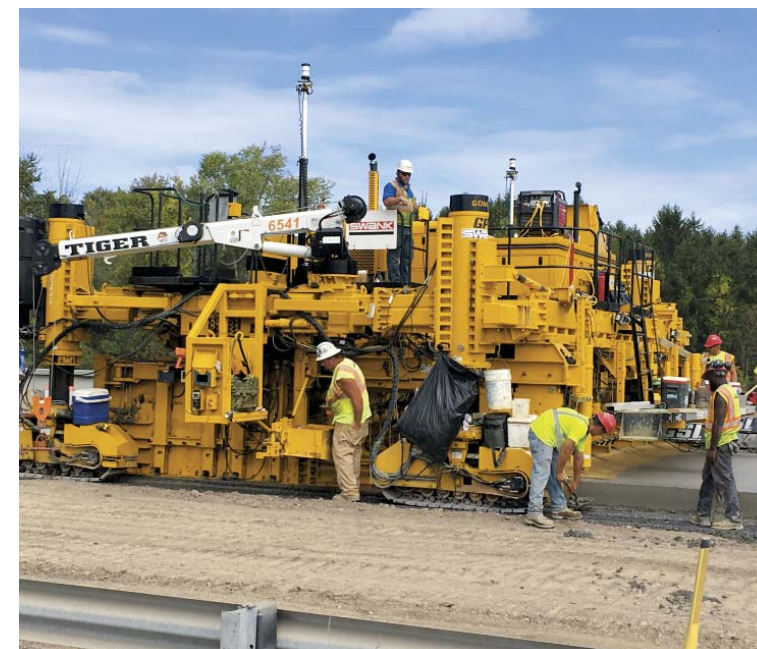
The GOMACO four-track GP3 is equipped with an IDBI attachment. The IDBI is an independent attachment that is self-contained, self-powered, and can insert transverse dowel bars into the pavement.
