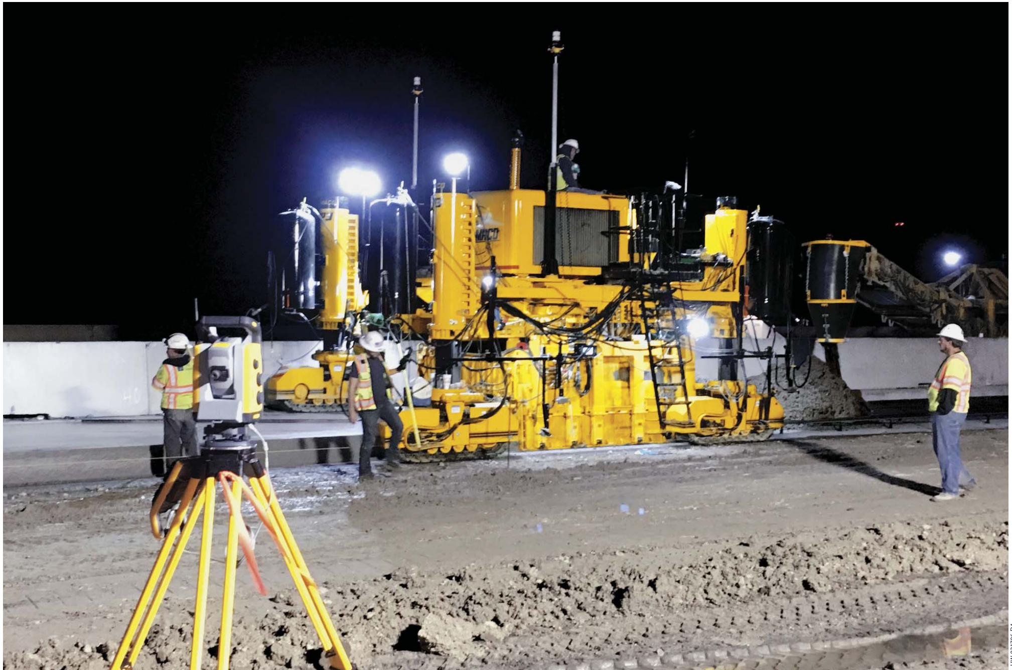
Night paving is only one of the challenges on this project. The four-track GP3 with 3D machine guidance slipforms ten feet (3.05 m) wide over continuous steel reinforcing, while the paver's left side tracks run within inches (millimeters) of the barrier wall.
