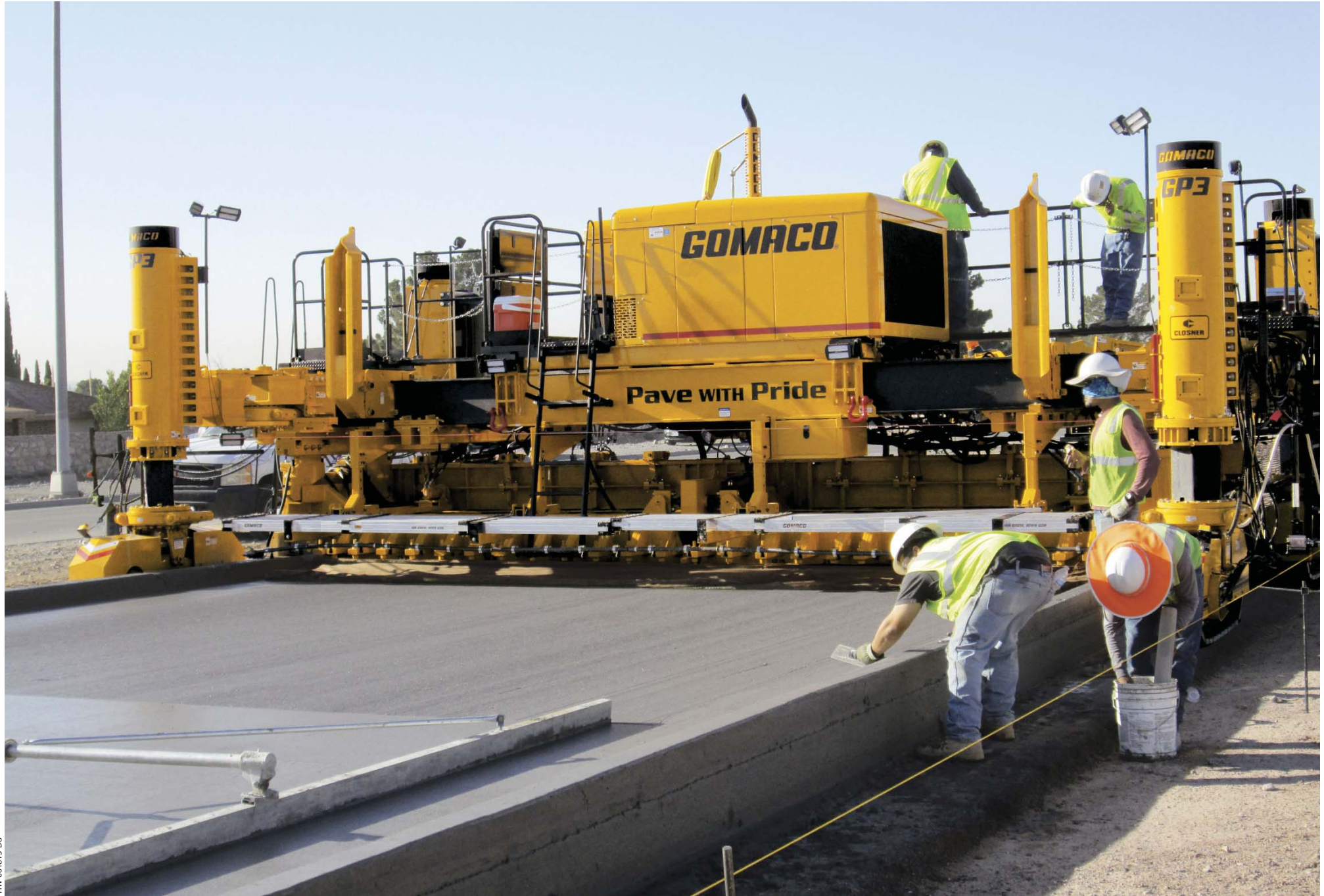
Equipped with a 5000 series paving mold, this GP3 four-track slipforms 26 feet (7.92 m) wide with integral curb on both sides of the slab.
