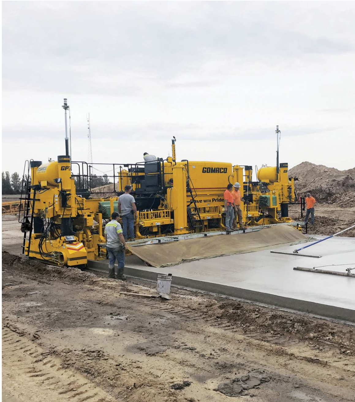
A two-track GOMACO GP3 slipforms a project with integral curb on both sides of the slab using 3D machine guidance. This GP3 is also equipped with GOMACO Remote Diagnostics (GRD), allowing for fleet management from a cell phone or laptop computer.
