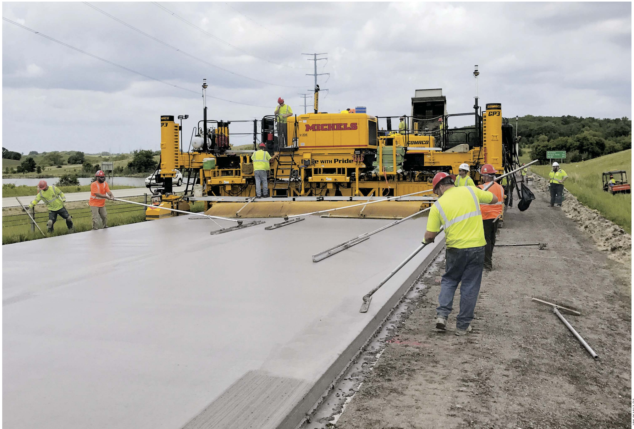
This GOMACO four-track GP3 is equipped with two 5400 series bar inserters to slipform this interstate project. The 5400 series bar inserter is rear loading for quick and easy accessibility.
