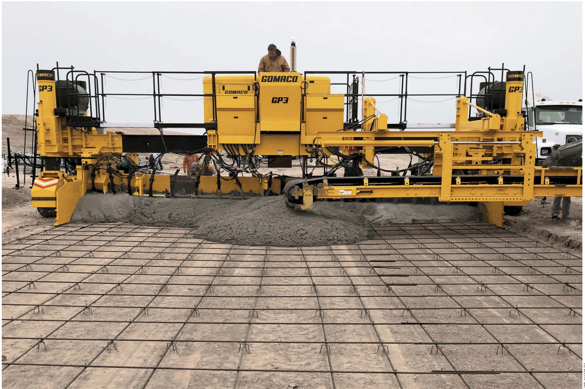
A special front mounted conveyor was added to this two-track GP3 for concrete placement. The ready-mix trucks were not able to get in front of the machine because of the steel rebar grid laid out on the grade, so the conveyor was added and the trucks discharged the concrete from the left side of the paver.
