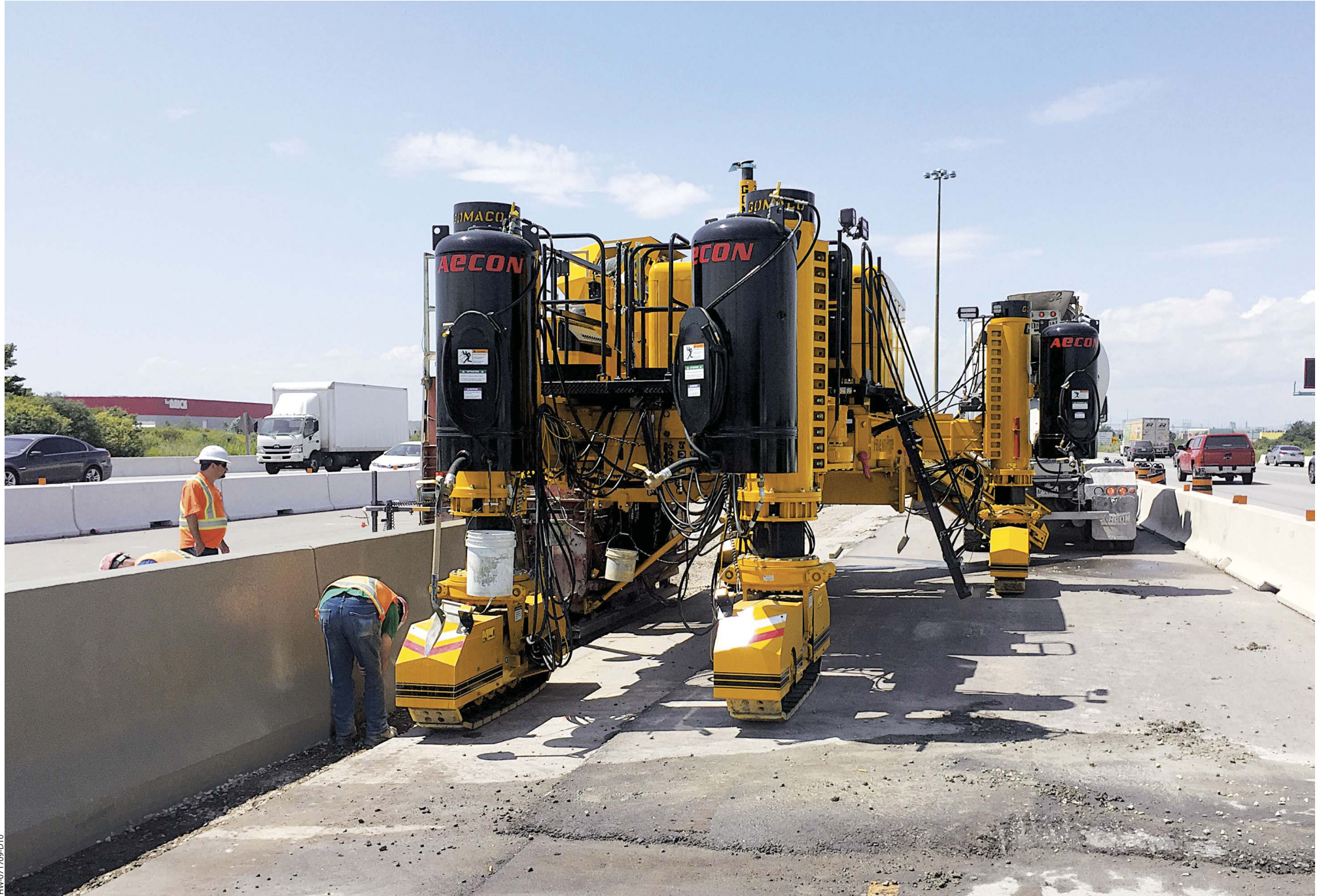
The four-track GP3 slipforms variable barrier with the mold sidemounted on the paver and the conveyor mounted on the endcar.
