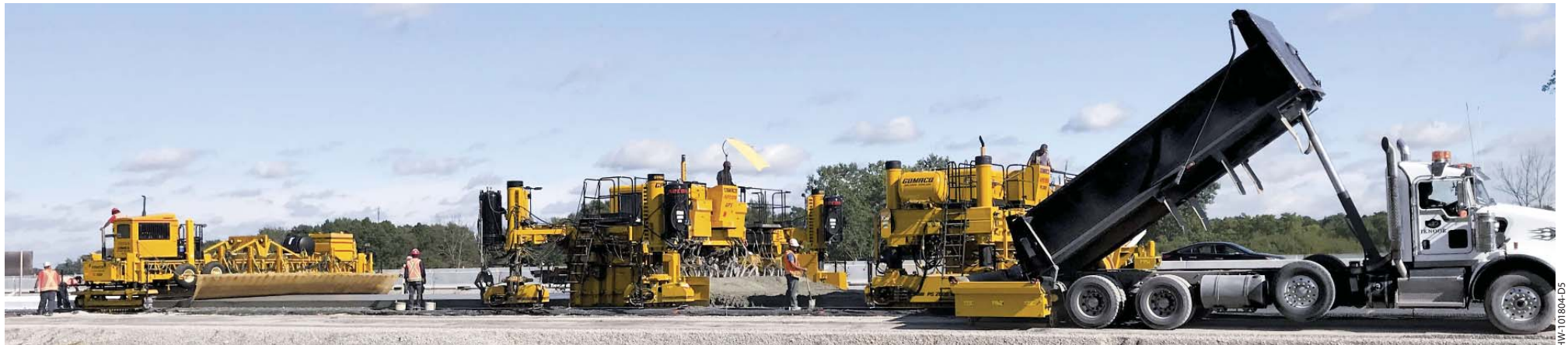
A GOMACO paving train consisting of the PS-2600 placer/spreader, GP3 four-track slipform paver, and the T/C-600 texture/cure work to complete a highway project quickly and efficiently. GOMACO's leg mounted water tanks are bottom filling and require no ladder to refill.
