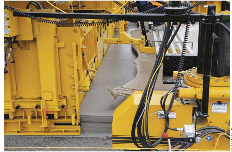
The GP3 with 5400 series mold produces a smooth, clean, and sharp edge or with keyway on this new roadway project for a commercial development.
