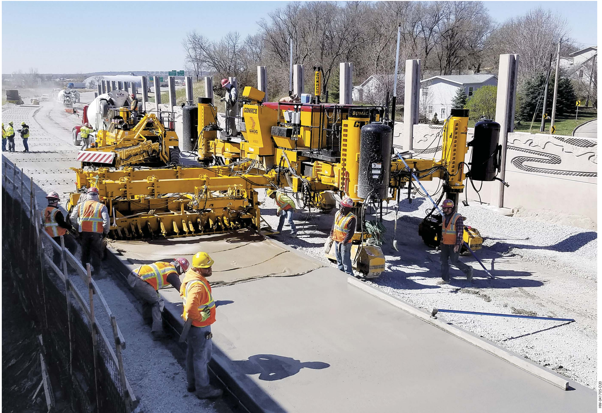
Minimum clearance is achieved when the GP3 is turned to transport mode with a sidemounted mold to slipform a 12 foot (3.66 m) section of interstate.
