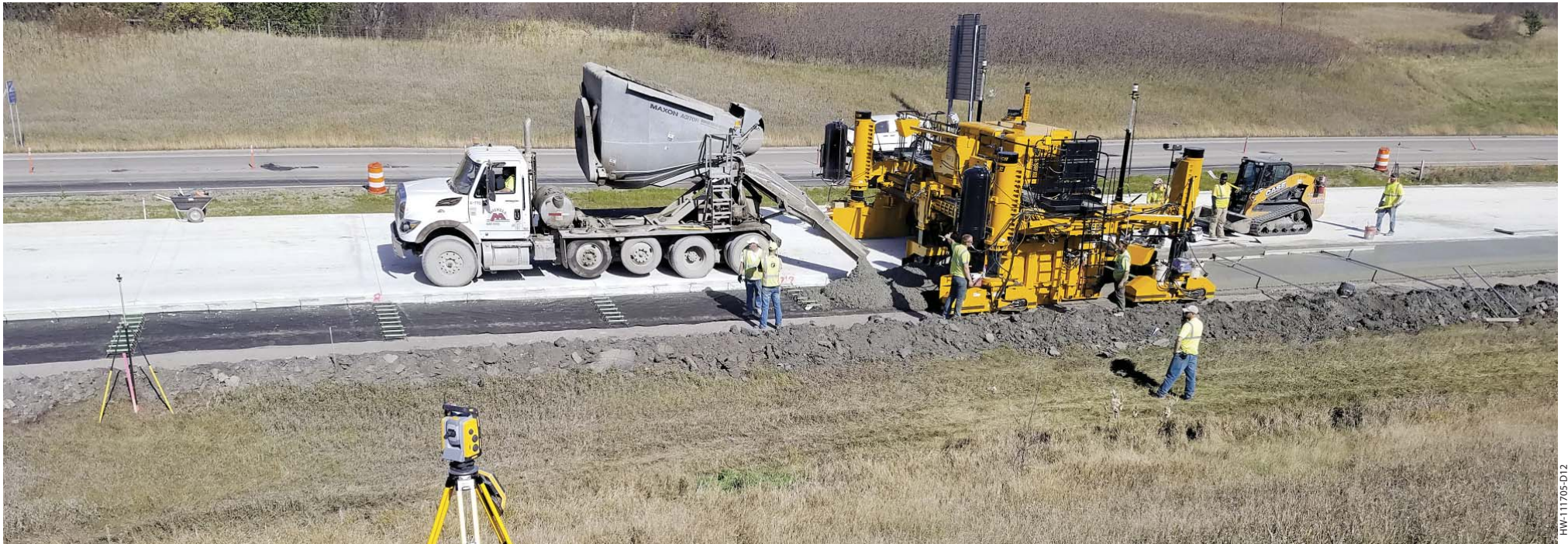
Using 3D machine guidance and the GOMACO G+ control system, this four-track GP3 slipforms a shoulder on an interstate project.
