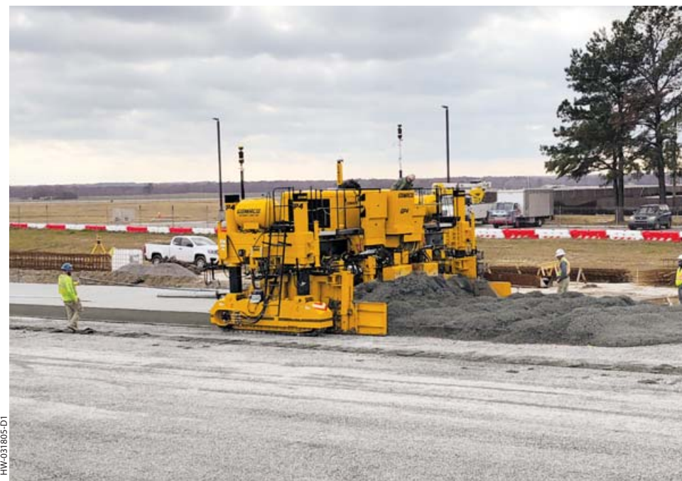
This GOMACO GP4 two-track slipform paver with 3D machine guidance slipforms an airport taxiway at 25 feet (7.62 m) wide, 22 inches (559 mm) thick.
