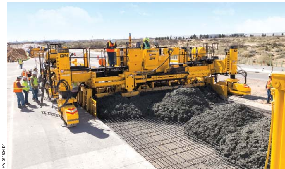
A highway expansion is efficiently accomplished with the GP4 four-track slipform paver.
