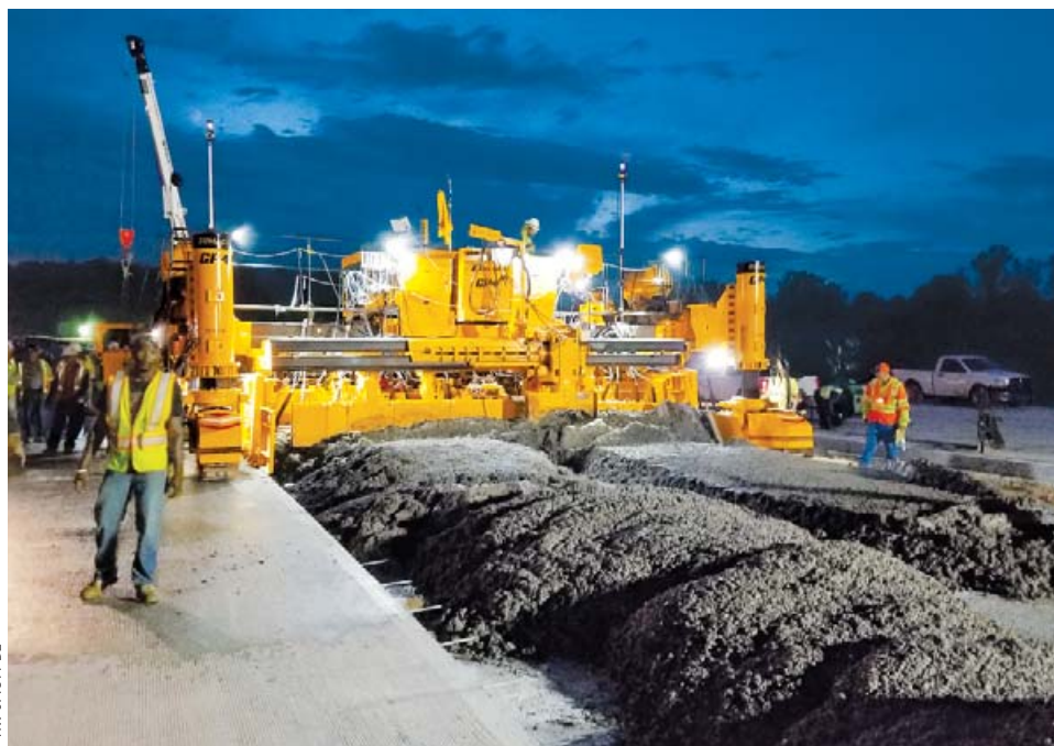
This four-track GP4 slipform paver is equipped with a telescoping spreader plow to evenly spread the placed concrete across the grade.
