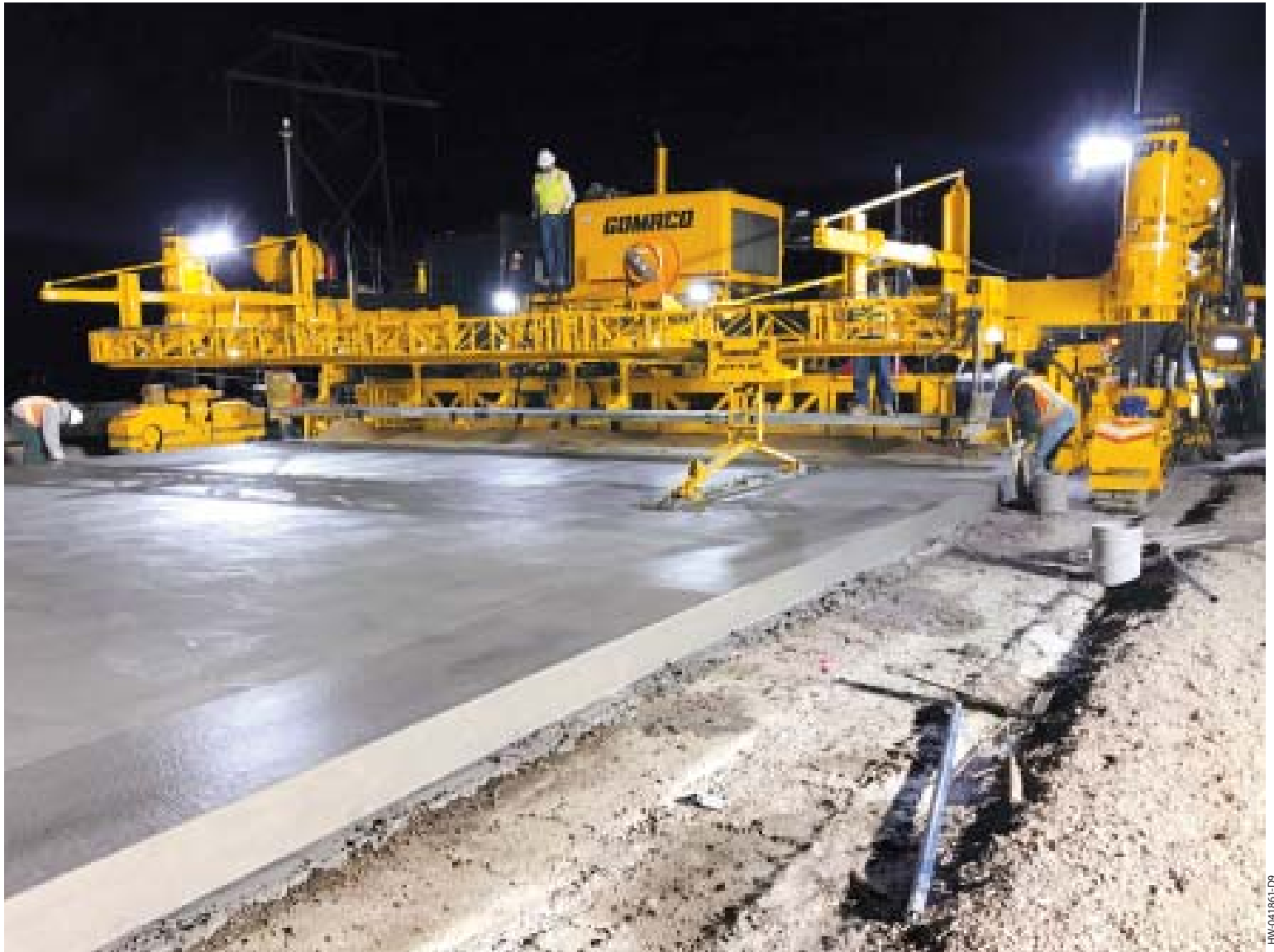
The GOMACO GP4, four-track, slipforms highway expansion at 38 feet (11.58 m) wide. The GP4 is equipped with the 5400 series paving mold, an Auto-Float®, and 3D machine guidance.
