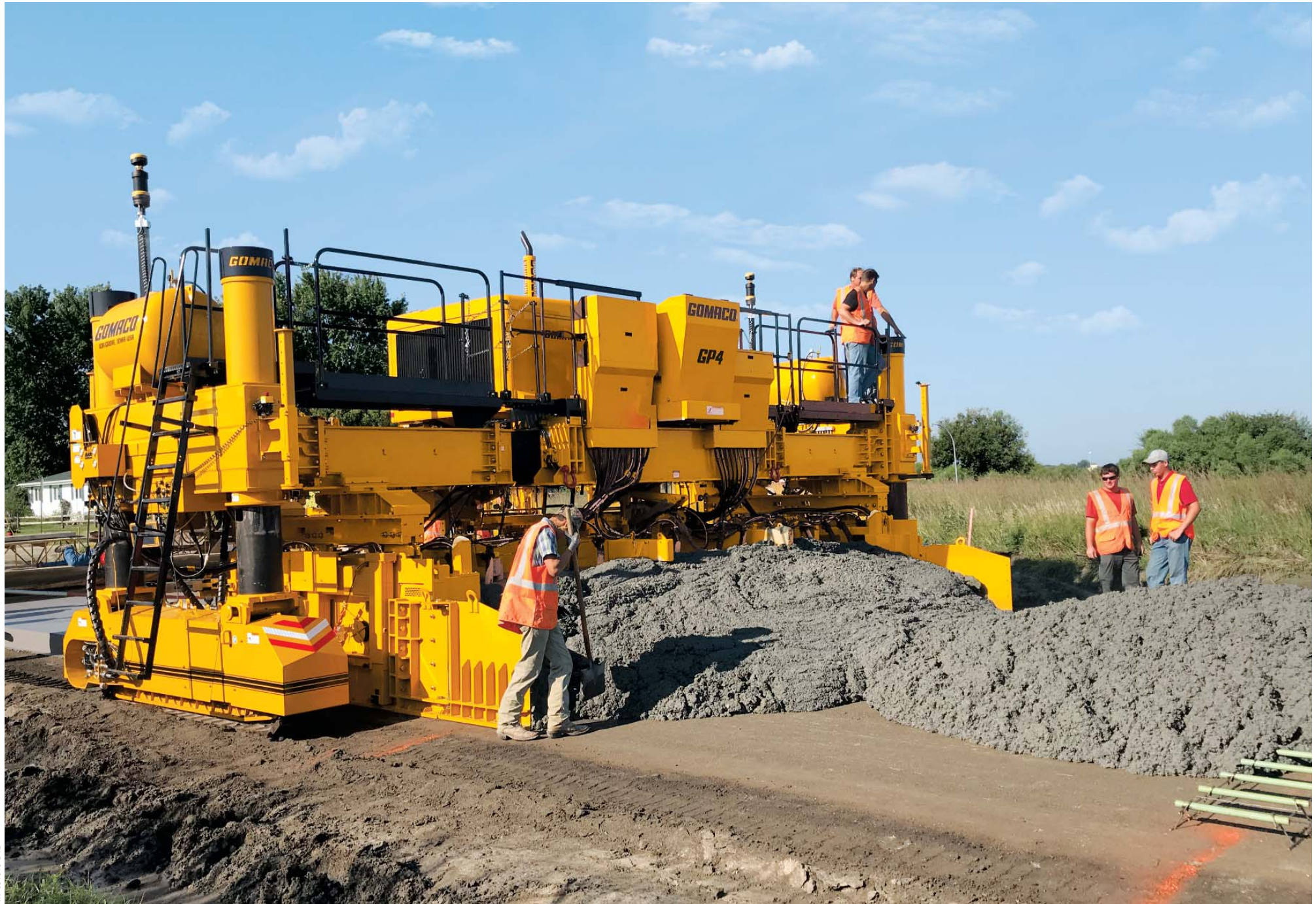
A two-track GP4 with a 5000 series open-front auger/strike-off mold and a 5400 series tie bar inserter slipforms a new street project using 3D machine guidance.
