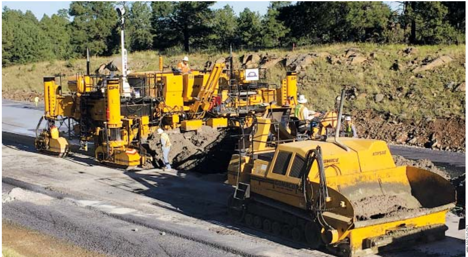
The GOMACO GP4 slipforms a 24 foot (7.32 m) wide section of interstate using 3D machine guidance. The GOMACO RTP-500 places the concrete in front of the paver.
