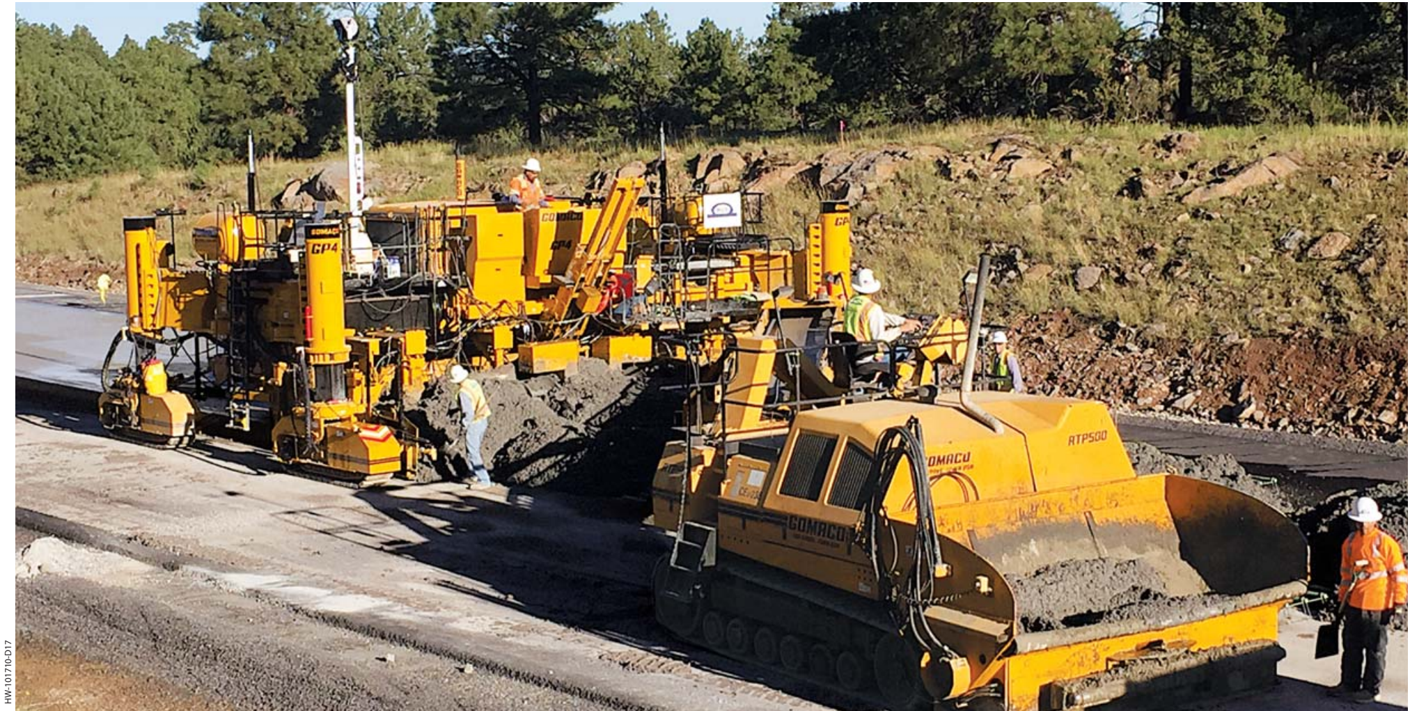
The GOMACO GP4 slipforms a 24 foot (7.32 m) wide section of interstate using 3D machine guidance. The GOMACO RTP-500 places concrete in front of the paver.
