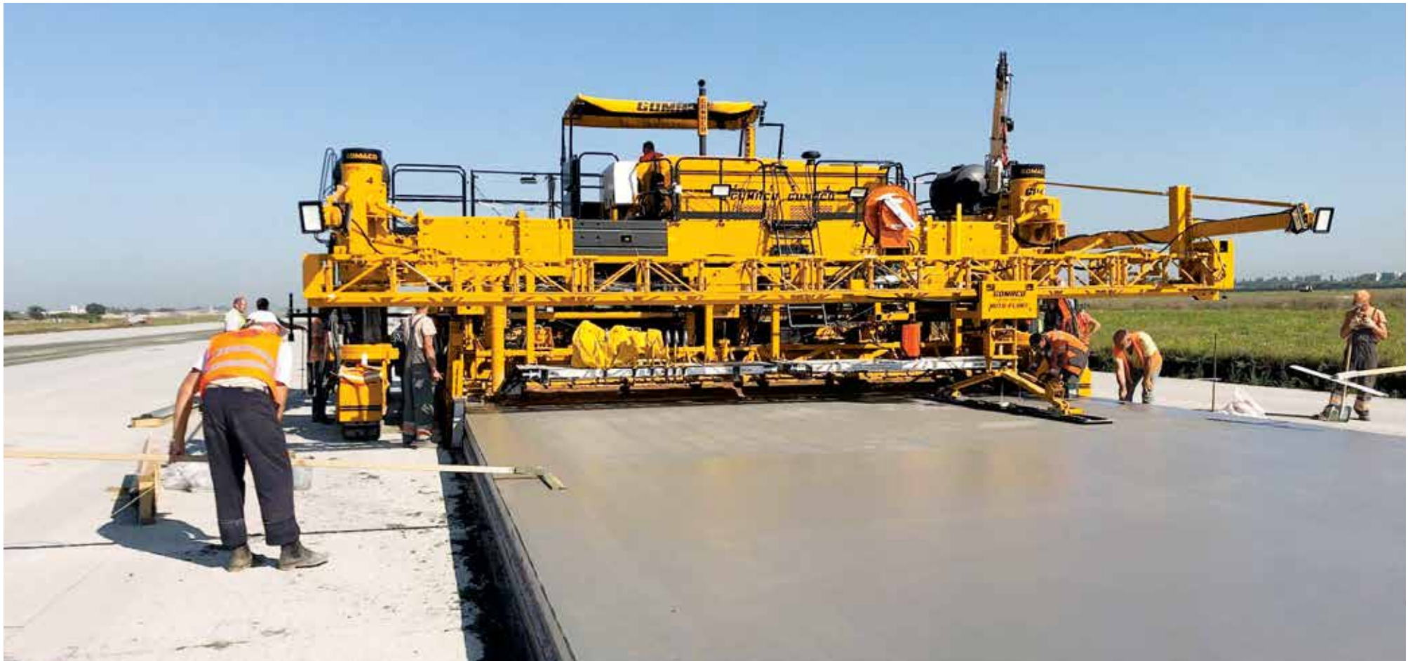
This GP4 slipform paver features a 5000 series mold with an Auto-Float ® to complete a smooth finish across this airport project.
