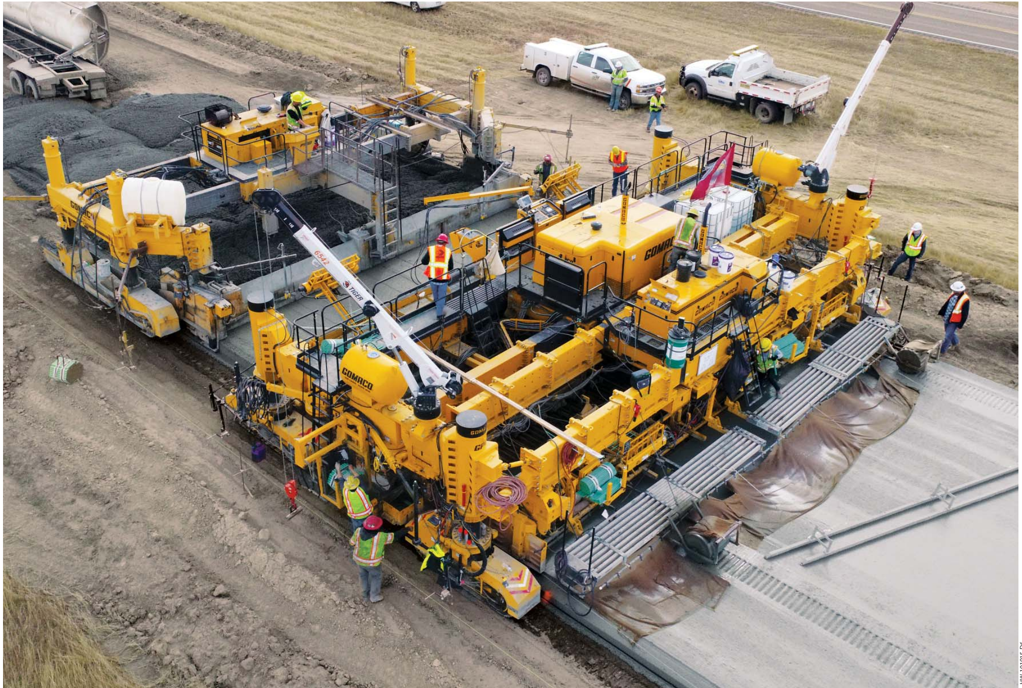
A GOMACO PS-60 spreads concrete ahead of the four-track GP4 equipped with an IDBI (Independent Dowel Bar Inserter) and two 5400 series tie bar inserters to place the dowel bars at DOT (Department of Transportation) specifications on this interstate project. The IDBI is an independent attachment that is self-contained, self-powered, and inserts transverse dowel bars into the pavement.
