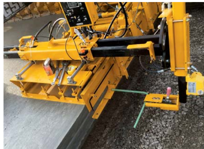
The two-track hydraulic powered bar inserter trails behind the mold and tracks.
