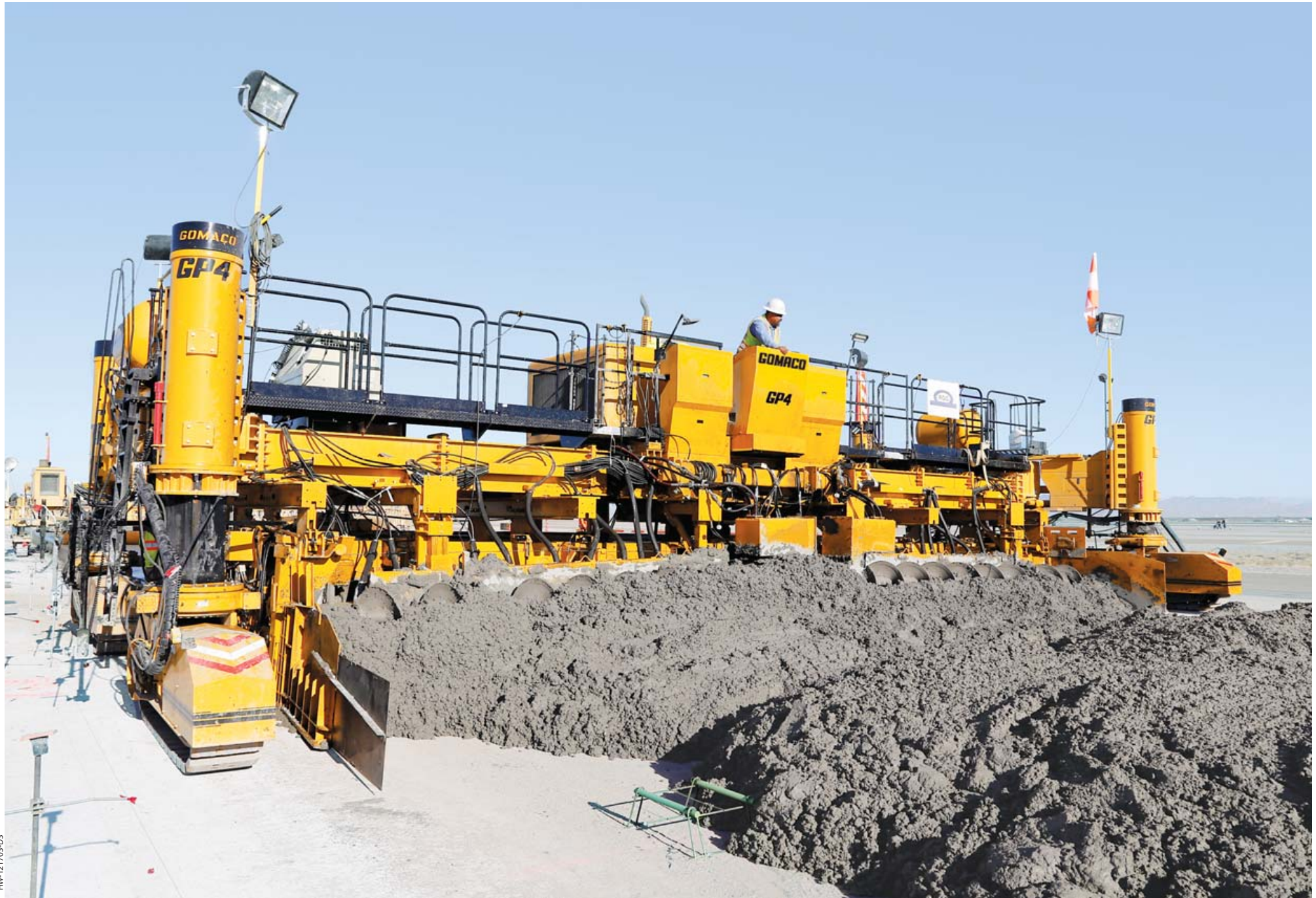
A new runway slipformed 37.5 feet (11.43 m) wide and 19 inches (483 mm) thick with the GP4 four-track featuring a 5000 series auger/strike-off to spread the concrete across the grade.
