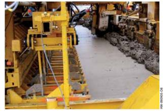
**5:** The DBI attachment's finishing process includes a tamper bar, unique oscillating straightedge, paving pan and stainless that follow the bar inserters and repair the scarring from the insertion process.
