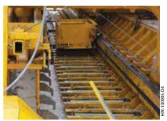
1: The bar loading trolley places a bar into each bar loading tray across the entire width of the new pavement.
