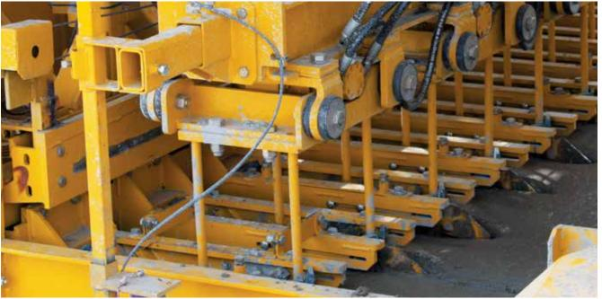
**3:** Vibration is applied to the forks on insertion to consolidate and close the concrete around the inserted bars. The vibration to the forks is variable, up to 7500 vpm. The paver never stops during the insertion process. GOMACO's exclusive computer-controlled smart cylinder technology provides the state-of-the-art system to maintain the accountability of the depth of the bars upon insertion into the slab.
