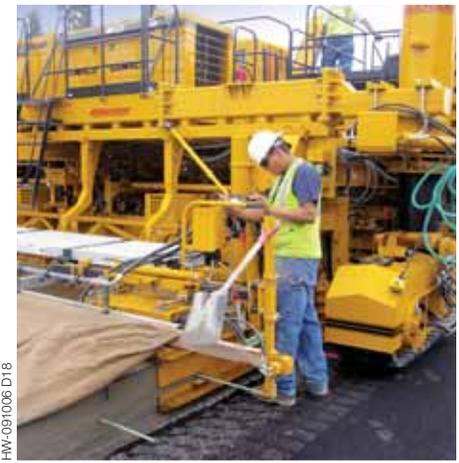
**4:** Once the tie bar has been inserted to the proper depth, a proximity switch will be activated, which will stop the vibration and switch the hydraulic valve to retract the hydraulic cylinder to make ready for loading the next tie bar for insertion.
