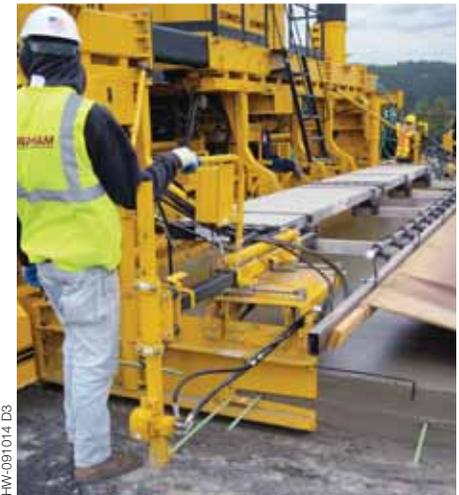
**6:** The operator then moves the inserter apparatus to the forward or home position with the attached handle and the process can begin again.
