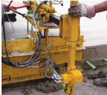
**3:** As the insertion process is started, the vibration will be turned on and the hydraulic cylinder will begin to insert the bar. The operator simply holds or guides the handle on the inserter to keep it stationary with the side of the slab as the paver continues to move forward.
