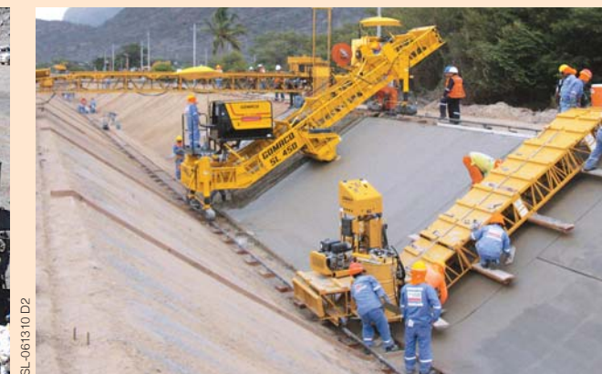
A new canal is under construction near Olmos, Peru. A GOMACO SL-450, RC Conveyor, and 2000 Series Spanit® are finishing the canal.
