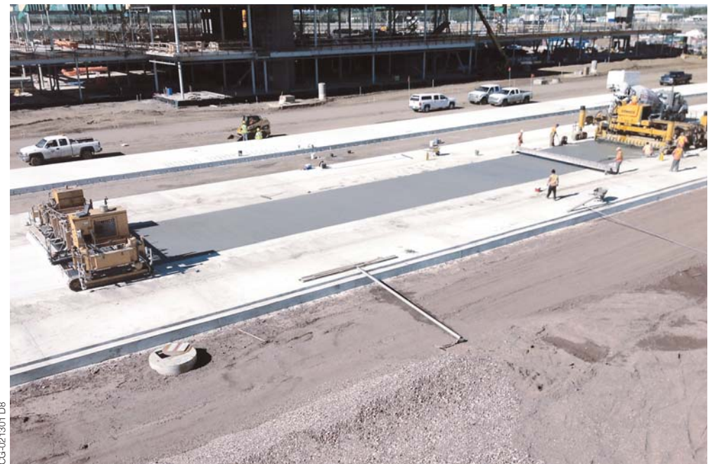
The Commander III slipformed the new apron in six paving passes. Each pass was 6.1 meters (20 ft) wide and 380 millimeters (15 in) thick.
