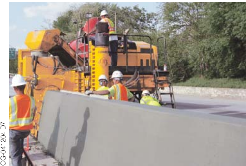
A three-track Commander III slipforms wall on the north end of the project.
