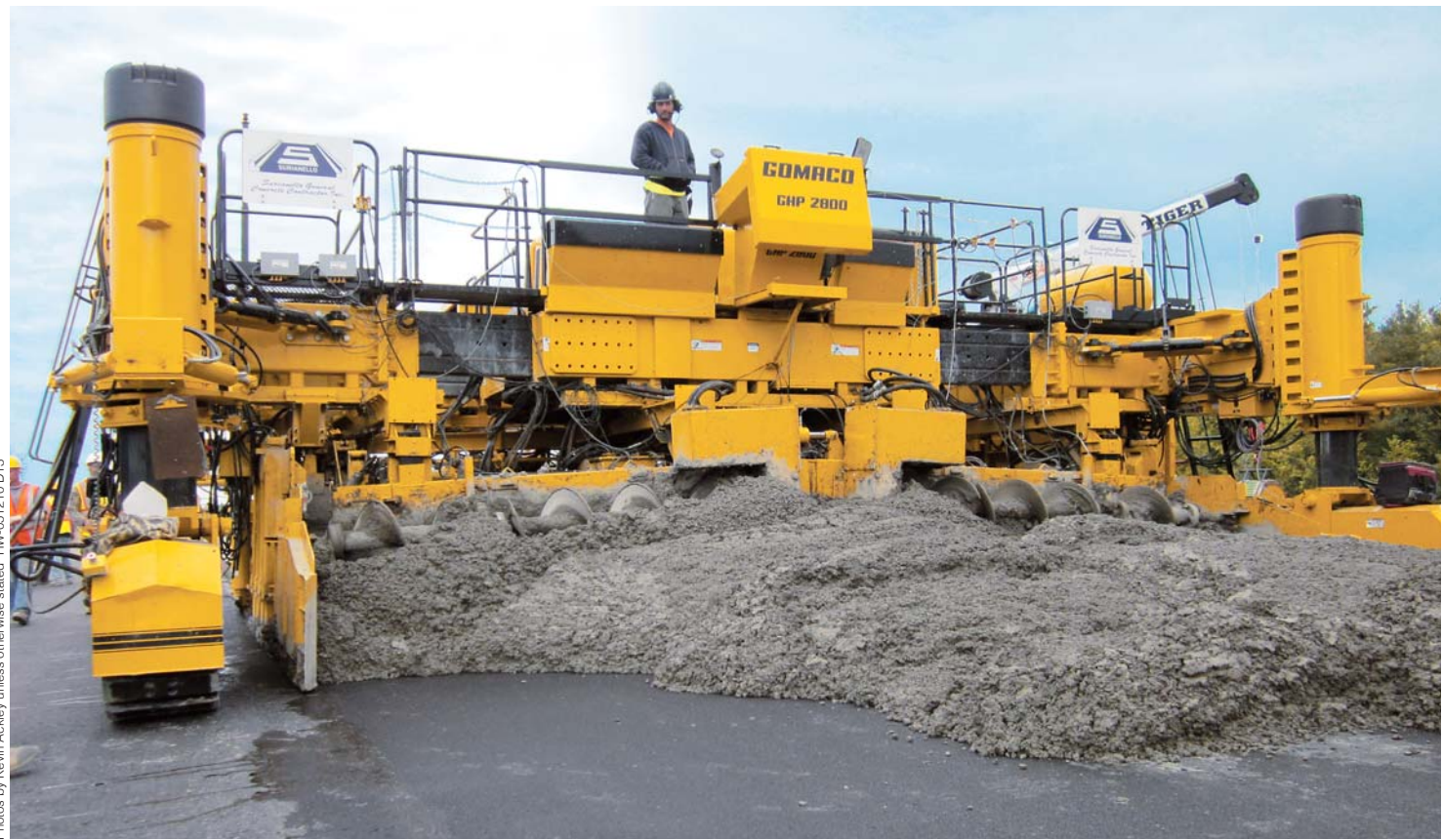
The new concrete overlay is part of a test section on Interstate 90. A GHP-2800 is slipforming the overlay on top of existing asphalt.
