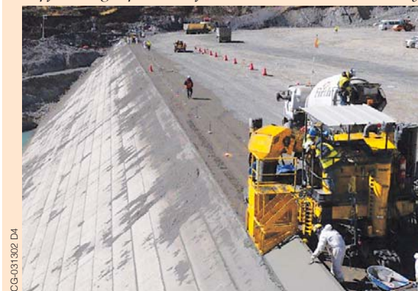
A Commander III on the Toromocho Dam Project is slipforming 4800 meters (15,748 ft) above sea level near Yauli, Junín, Peru.
