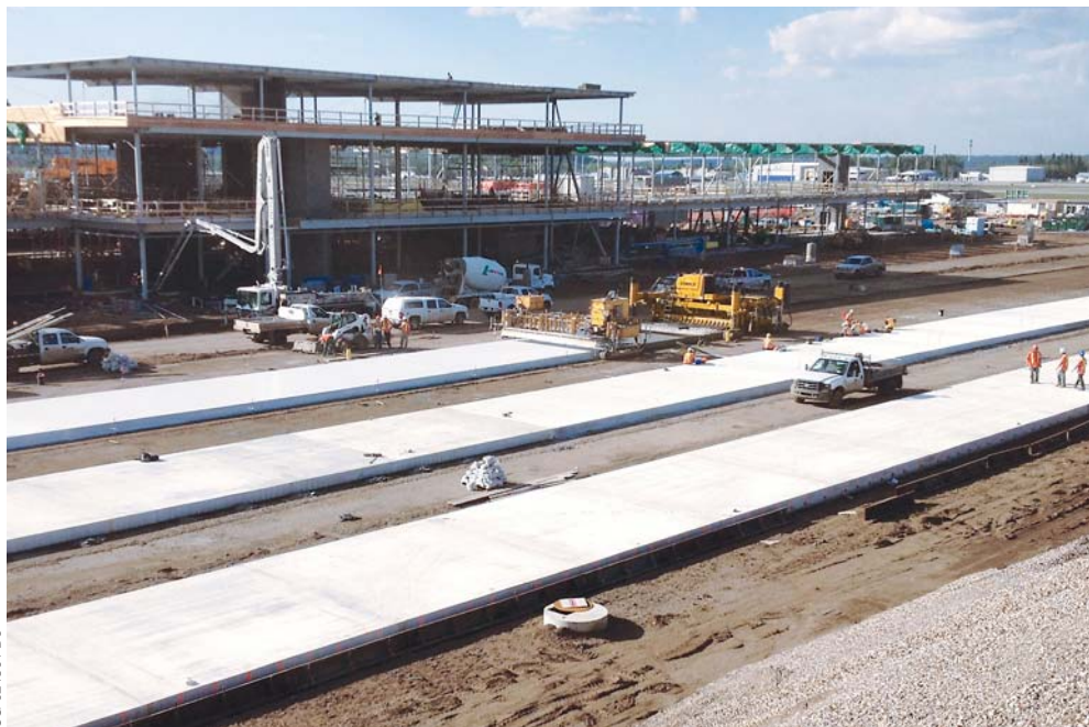
Proform Concrete Services Inc., used their GOMACO four-track Commander III to slipform an apron next to the new terminal building at the airport.
