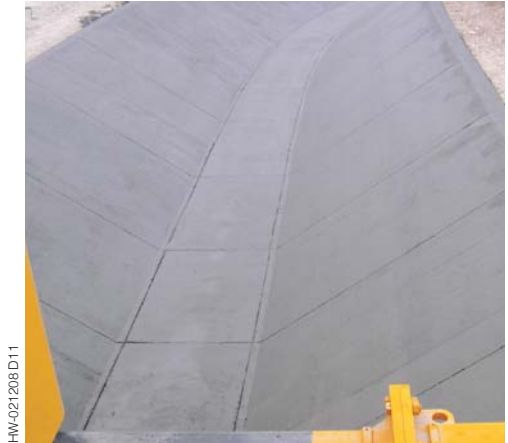
The operator's view of the canal shows the GP-2600 paver leaving a smooth finish.
