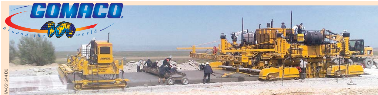
A GOMACO four-track GP-4000 with Leica 3D stringless control and a T/C-600 texture/cure machine is slipforming a portion of the New Silk Road near Shymkent, Kazakhstan.
