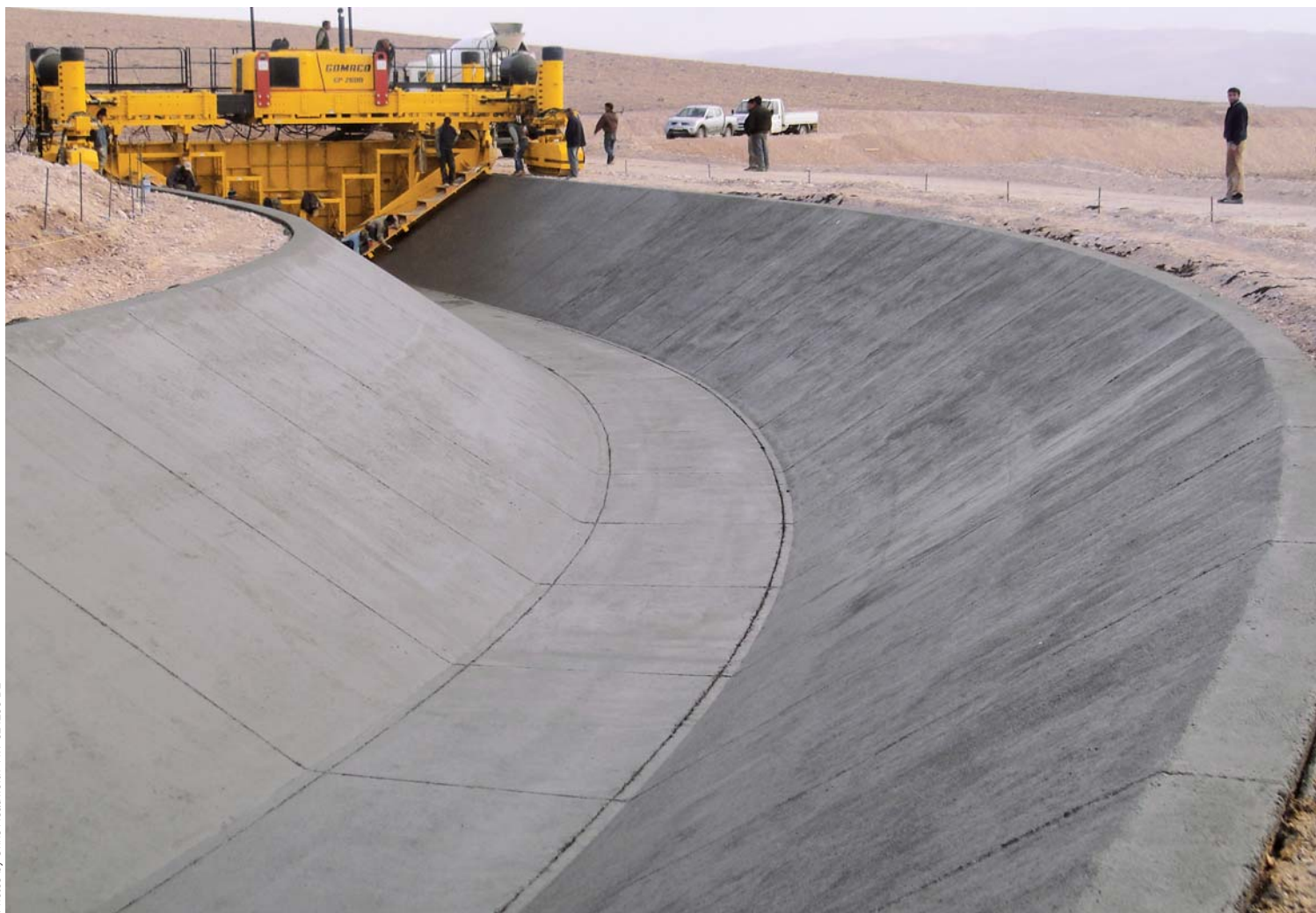
Fernas Construction and Trade Corp. slipforms the new Batman Canal in a single pass with their GOMACO four-track GP-2600 paver.
