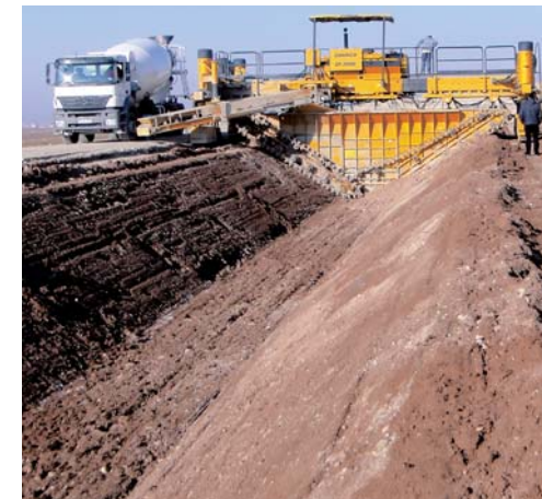
Fernas Construction and Trade Corp. slipforms the new Batman Canal in a single pass with their GOMACO four-track GP-2600 paver.
