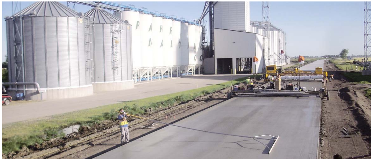
The paving on the project was the smoothest concrete pavement ever constructed in the state with an IRI of 38.6 before corrective action.
