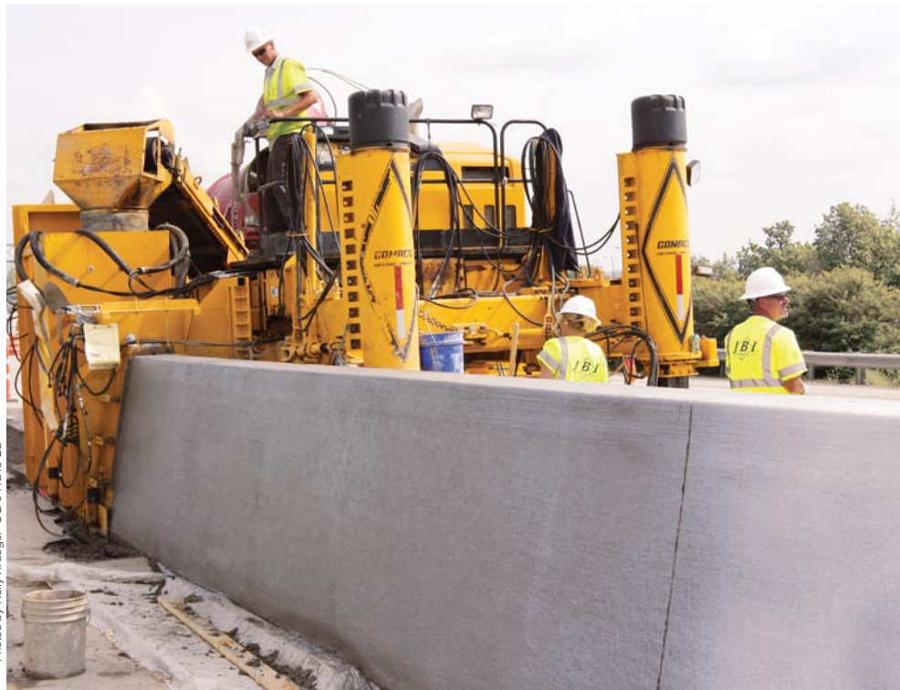
JBI Construction had their entire company and three of their GOMACO slipform pavers at work on the project, including their four-track Commander III.
