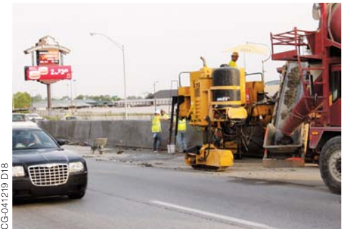
The third barrier machine on Louisville’s I-65 was a three-track GOMACO GT-6300.
