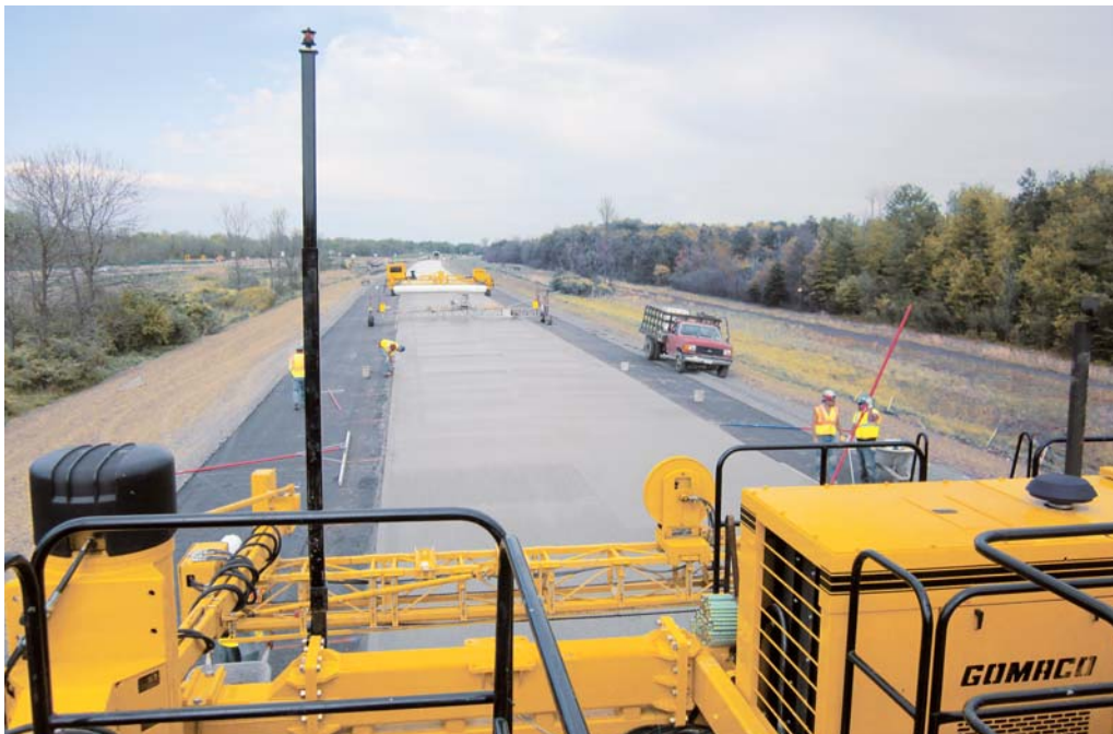
A GOMACO T/C-600 texture/cure machine followed the paver and applied a longitudinal tine and white spray cure.
