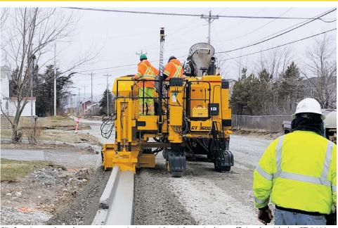
Slipforming curb and gutter in an existing residential area is done efficiently with the GT-3600 equipped with 3D machine guidance. The ability to block out existing driveways on-the-go allows for less follow up work.
