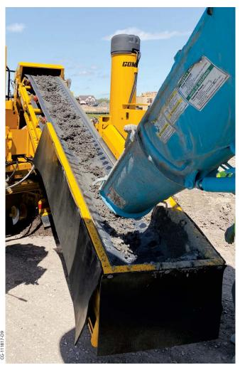
The 16 foot (4.88 m) long, 24 inch (610 mm) wide conveyor can move the concrete into the hopper at a speed of up to 284 feet per minute (86.6 mpm).
