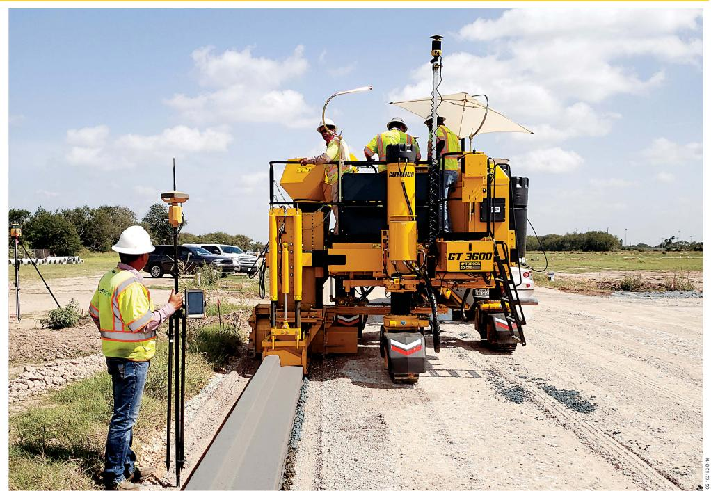
An 18 inch (457 mm) curb and gutter is slipformed using 3D machine guidance by the Xtreme GT-3600 in a new residential development.
