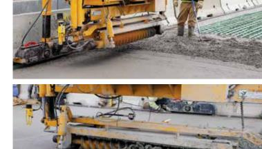
The 5.7 foot (1.74 m) long auger can advance as much as four feet (1.22 m) in a single pass.
