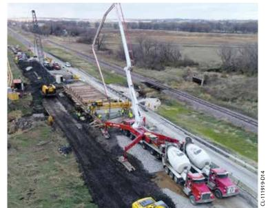
Two ready-mix trucks feed a concrete pump providing the C-450 and high-production screed with a constant supply of concrete to finish this 21 inch (533 mm) deep bridge project.
