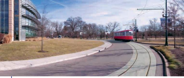
To minimize impacts to the Delmar and DeBaliviere roadways and vehicular traffic that will ultimately share the road with the trolley, the team is designing a shallow track slab allowing the rail and pavement to be flush and thereby eliminating safety hazards for both cars and pedestrians. A number of other elements will minimize roadway impacts and enhance safety for vehicles, pedestrians and trolley passengers.
