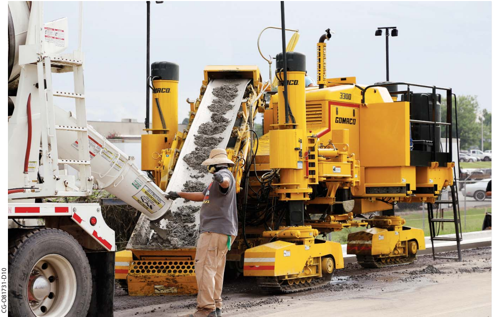
A 20 foot (6.1 m) folding conveyor to load the hopper is available on the GOMACO 3300. The conveyor can be positioned for either right-side or left-side slipforming. The conveyor folds to reduce the transport length of the paver.
