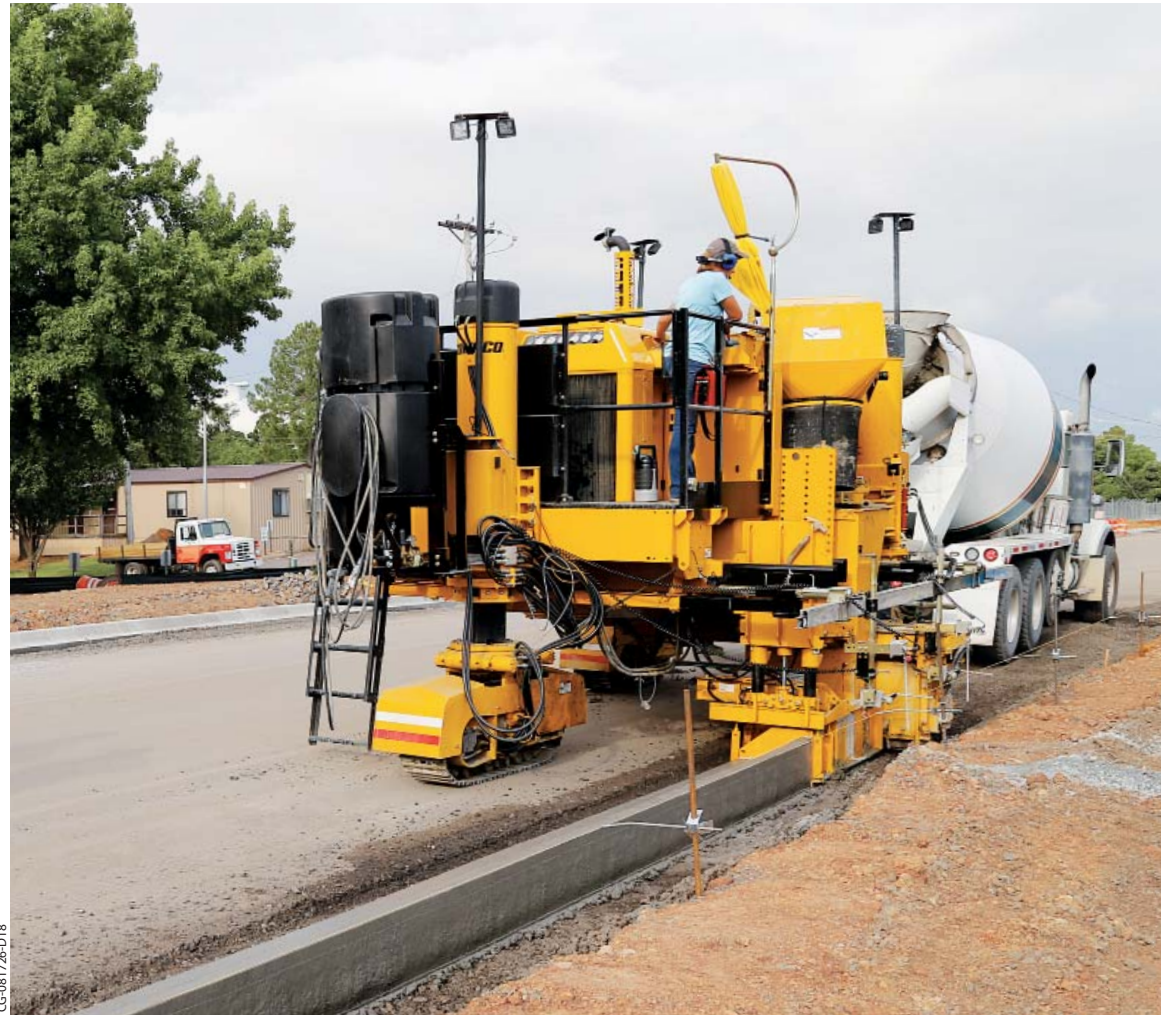
The hydraulic sideshift and lift on the 3300 allows the mold to easily slipform curb and gutter below the existing grade on rehab projects.
