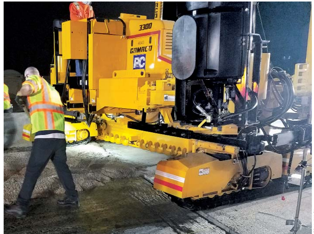
A GOMACO 3300 with a special mold paves a 0.75 inch (19 mm) thick polymer overlay on a bridge.
