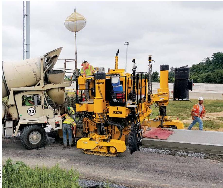
A GOMACO 3300 with an undermounted mold and 3D machine guidance slipforms a highway ramp eight feet (2.44 m) wide, 12 inches (305 mm) thick. The 3300's tracks are turned 90 degrees in the transverse position to accommodate the undermounted mold.
