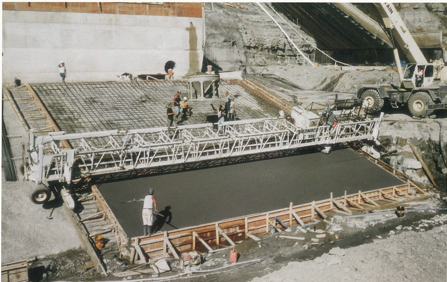
Photos courtesy of Getkate Construction Ltd. SL-100001-D #1
