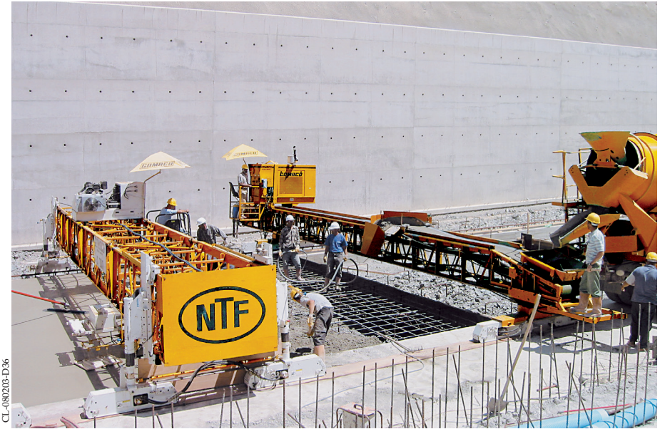
An RC Conveyor places the concrete ahead of the cylinder finisher.
