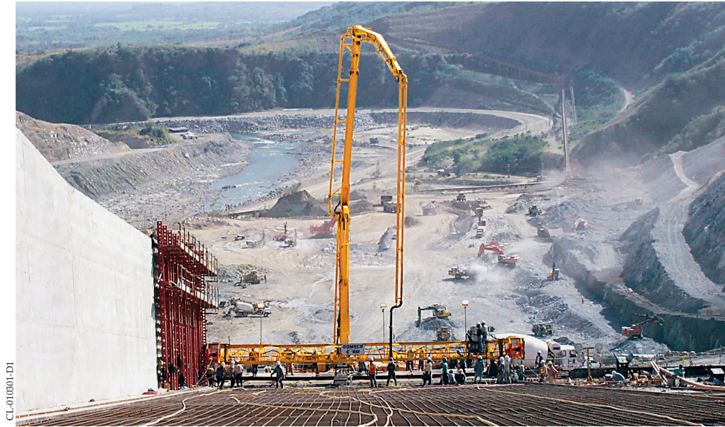
This GOMACO machine paves a spillway on the San Roque Dam in San Roque, Philippines.
