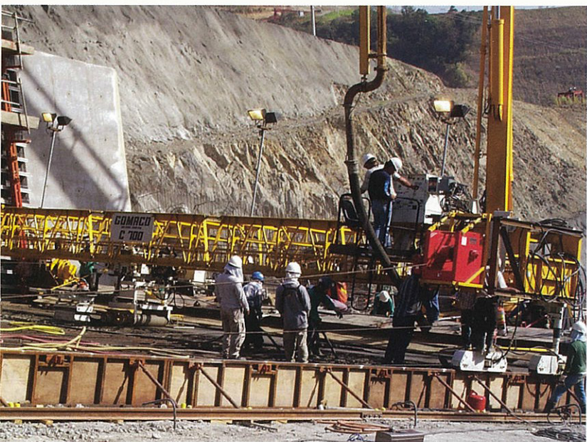
The C-700 finishes a portion of the spillway. Some sections had slopes with 27 percent inclines.
