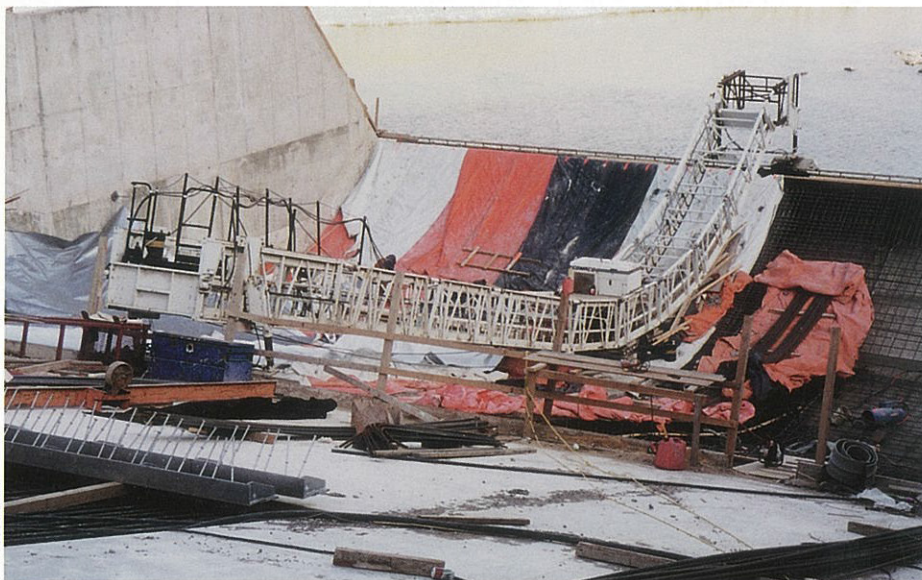
The flip bucket was poured longitudinally, however the slope and all the chute slabs were poured transversely at a 3:1 and 5:1 slope.
