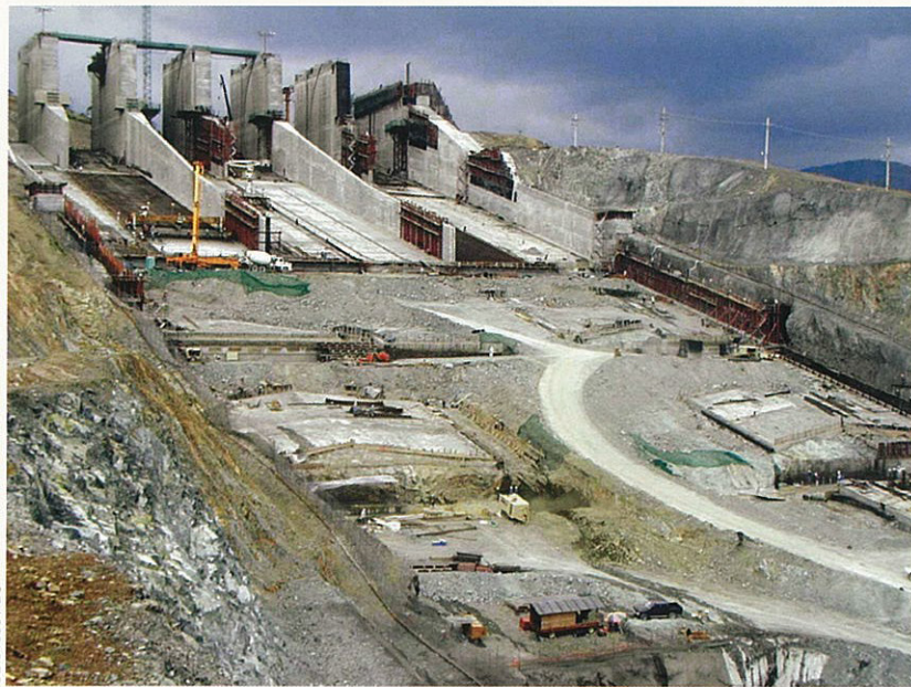
The C-700 finishes an upper section of the spillway while excavation and other work is in progress further below.
