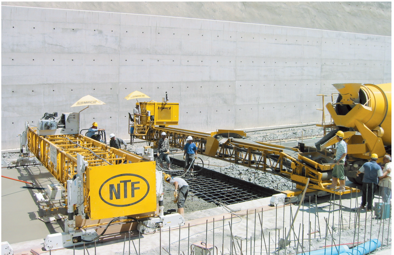
NTF Construction & Trading Ltd. continue to work with their GOMACO C-700 finisher on a spillway project in Dalaman, Turkey.
