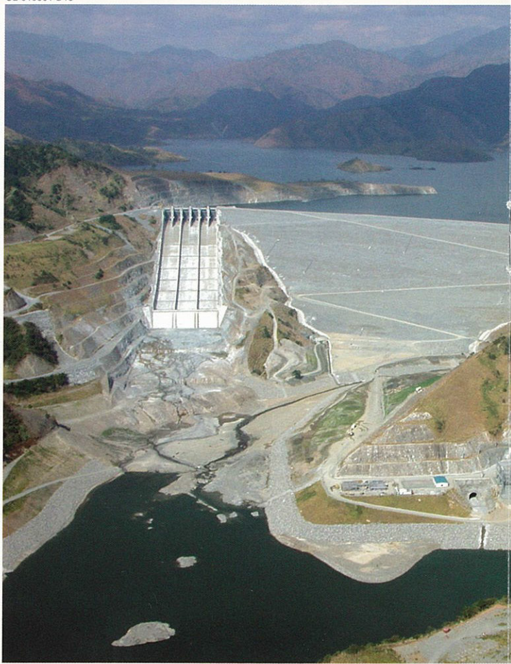
The San Roque Dam is a 656 foot (200 m) high embankment dam in the Philippines. Its spillway, in the upper left of the photo, is 1722 feet (525 m) long.
