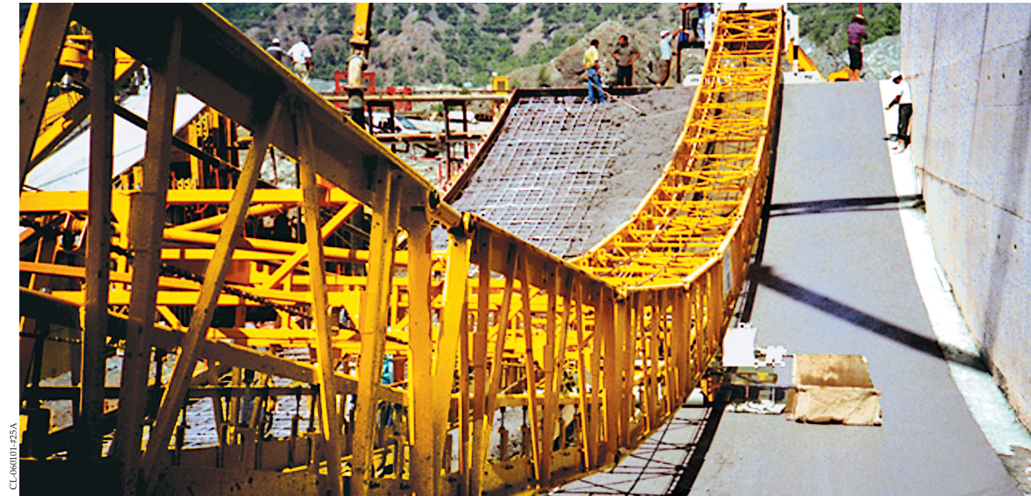
This GOMACO machine paves a spillway on the San Roque Dam in San Roque, Philippines.
