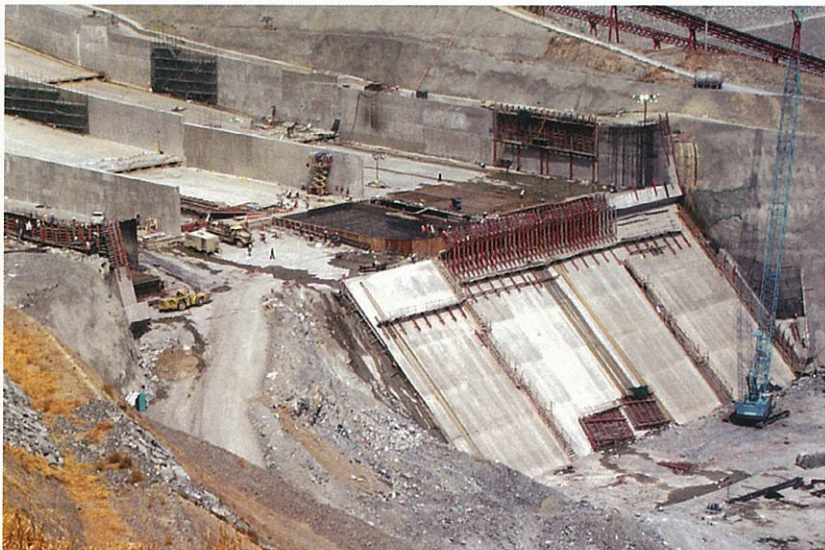
The spillway's flip bucket has a 70 foot (21 m) drop to dissipate the force of the water flowing down the chutes.
