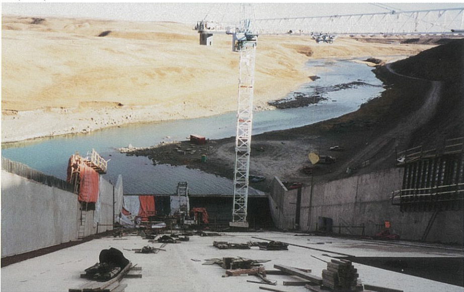
A view down the spillway and into the flip bucket. Concrete had to be placed in front of the C-700 with a crane and bucket. The 5076 psi (35 MPa) mix couldn't be pumped.
