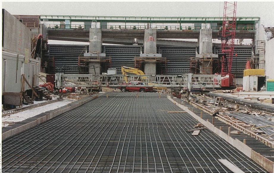
The concrete slab averaged two feet (.6 m) thick with production averaging 246 to 262 feet (75 to 80 m) an hour.
