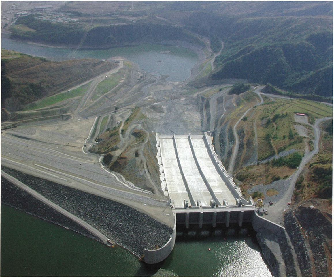
A view from behind the spillway shows the nearly completed spillway in late December 2002. The spillway's three sections were each 98 feet (30 m) wide.
