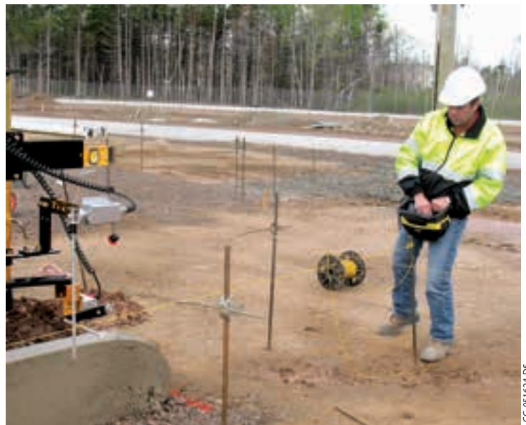
The remote has safety features like the emergency stop button and the alert horn located in convenient locations for quick access. There are also tilt and impact sensors in the remote for an automatic safety stop.
