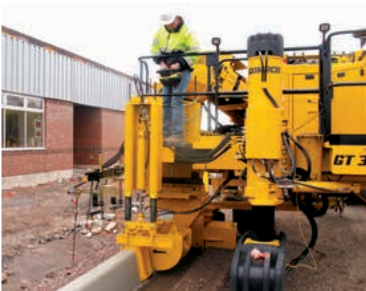
The operator can work from the operator's platform or on the ground with the G+ remote in order to get the best view of the paving operation.
