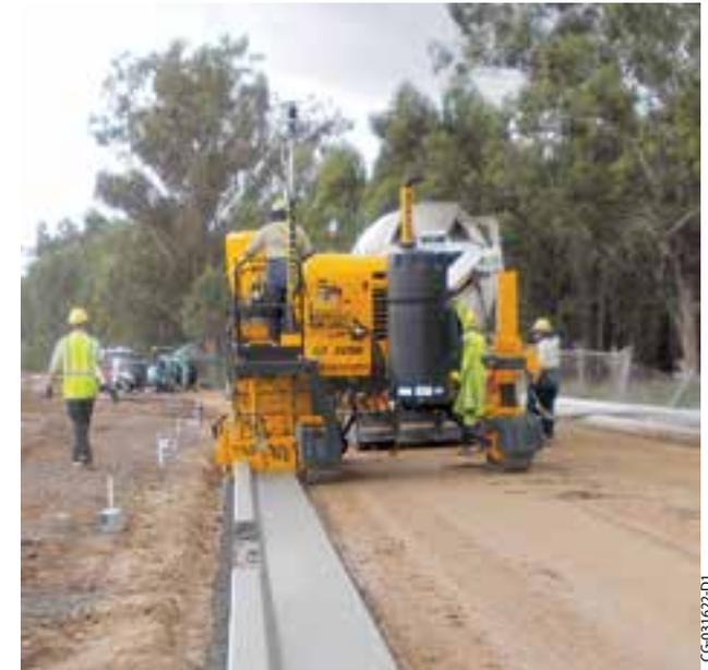
The GT-3200's mold can be equipped with an optional curb depressor when slipforming curb and gutter.
